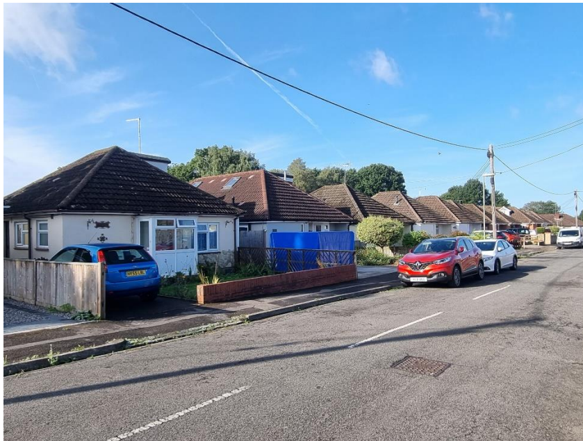
Neighbouring dwellings along Horton Way. A number of these properties have had extensions and roof conversions.
