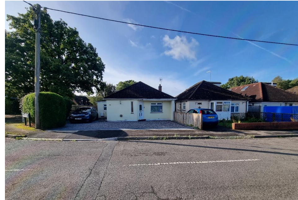
30 Horton Way and neighbouring property street view.
