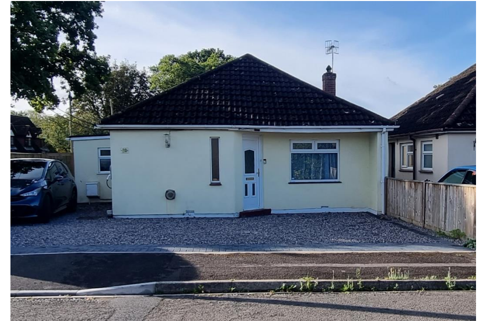
Front/ North, street facing elevation, with off street parking.
