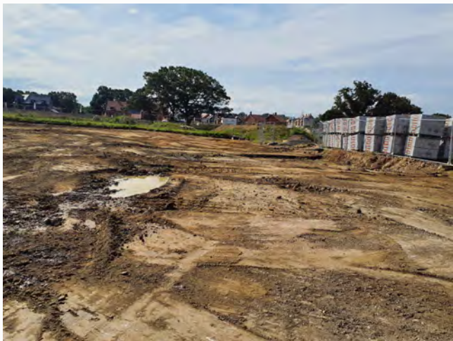
DescriptionReduced Dig Area A
