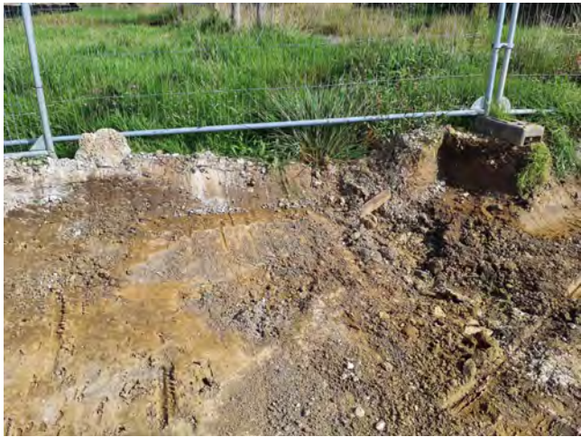
DescriptionReduced Dig Area A
