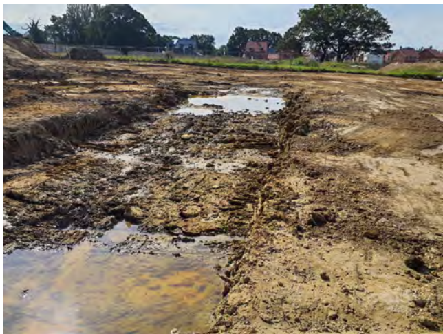
DescriptionReduced Dig Area A
