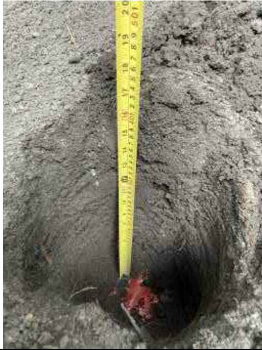
Photograph 5 HP302 Validation Pit
