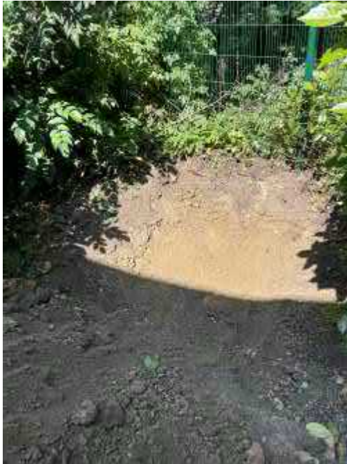
Photograph 7 VP102 Excavated to 450mm bgl
