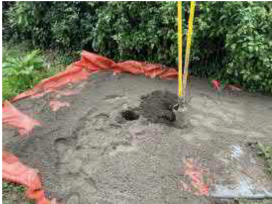
Photograph 3 VP101 with clean cover system installed
