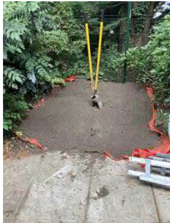
Photograph 8 VP102 with clean cover system installed
