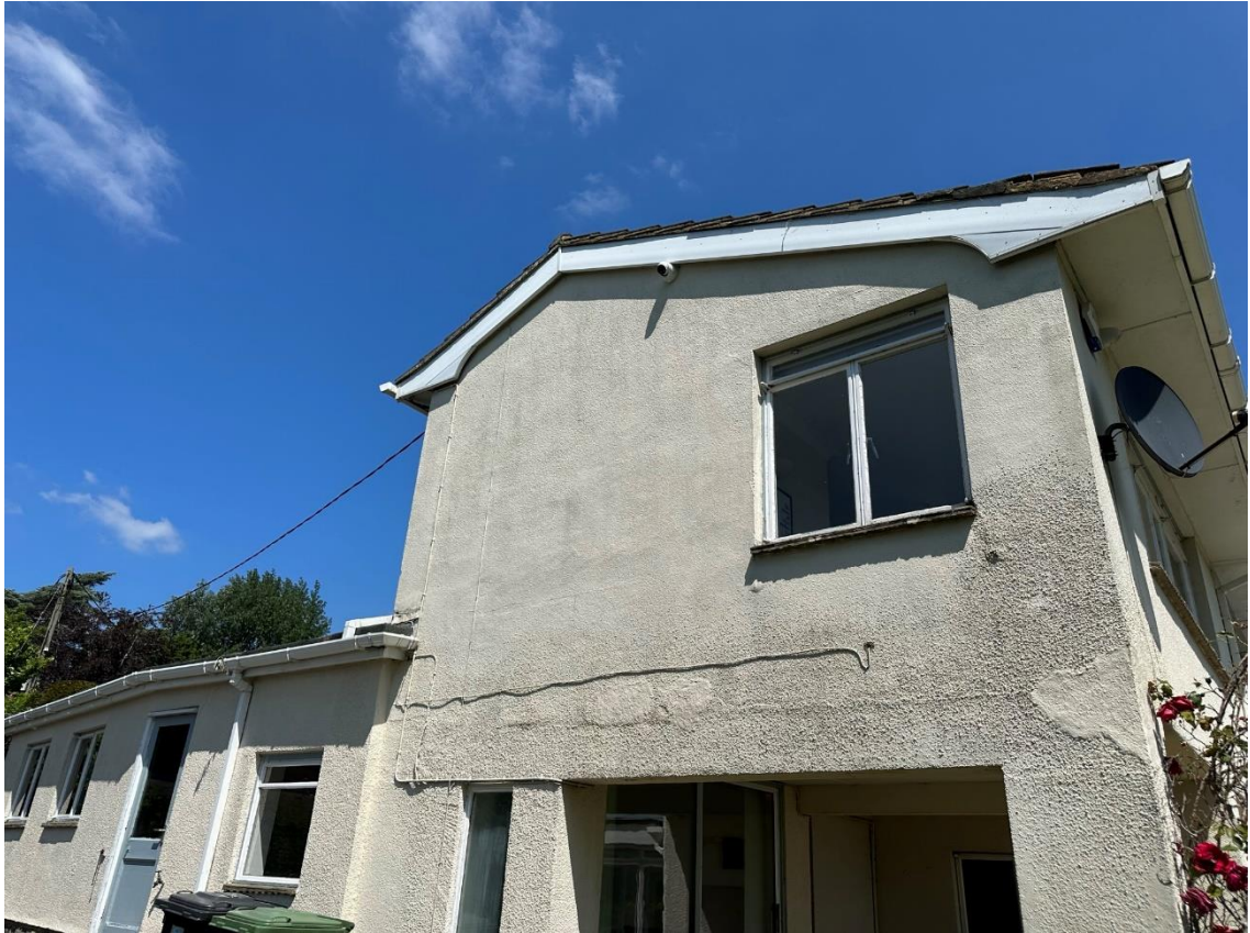
Photo 3- Close up of eaves showing tight structure
