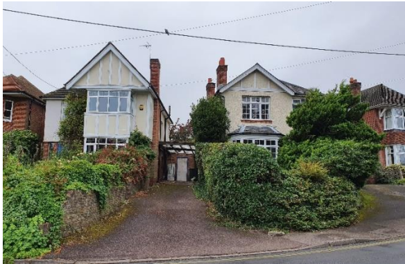
Figure 1: Front elevations of 13 & 15 Satchell Lane. The proposed excavation to road level (removal of 150 tonnes of soil) to enlarge the parking area; and the ground floor extension adjacent to subsidence at 15 Satchell Lane. Moreover, the lack of meaningful front garden and the predominance of hard surfaces would not only result in a loss of habitat (front and rear gardens) but is at variance with the natural existing contours and will create an unduly harsh environment that is out of character with the street scene/visual landscape.
