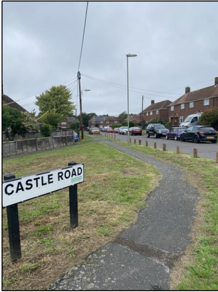
Photograph 4: Castle Road Footways
