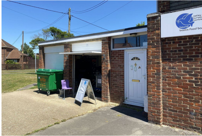
Figure 14. Front elevation of the garage attached to 30 Queens view (taken June 2022).
