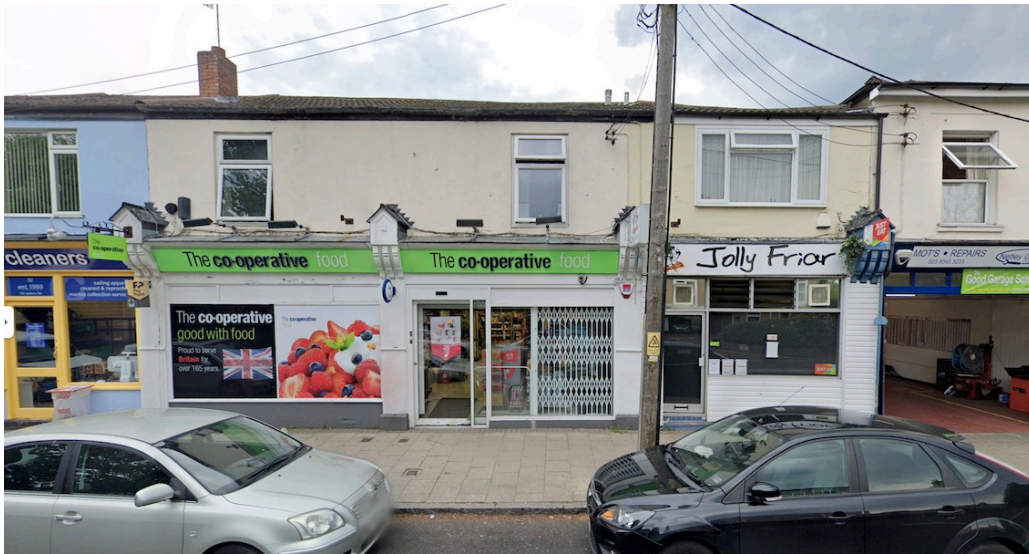
Figure 12: 33, 34, 35 Victoria Road showing removal of historic entrances
