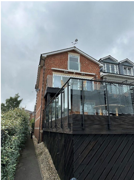
Rear of the house
