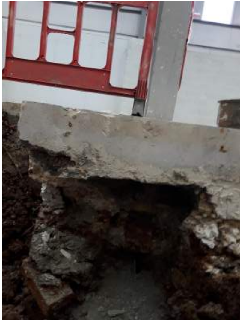
Photo 9: Image of TP07 under steel.
