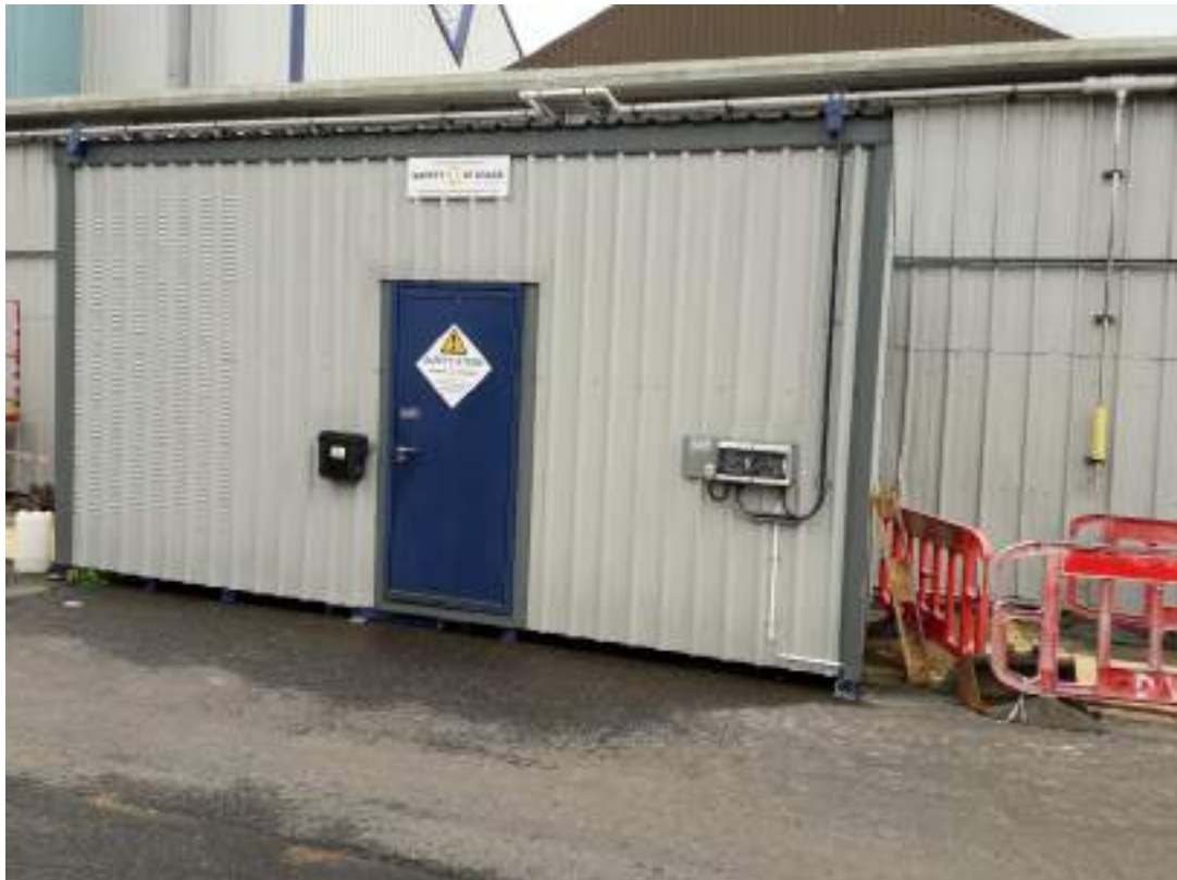
Photo 1: Image of locked storage building at north west end of commercial building.
