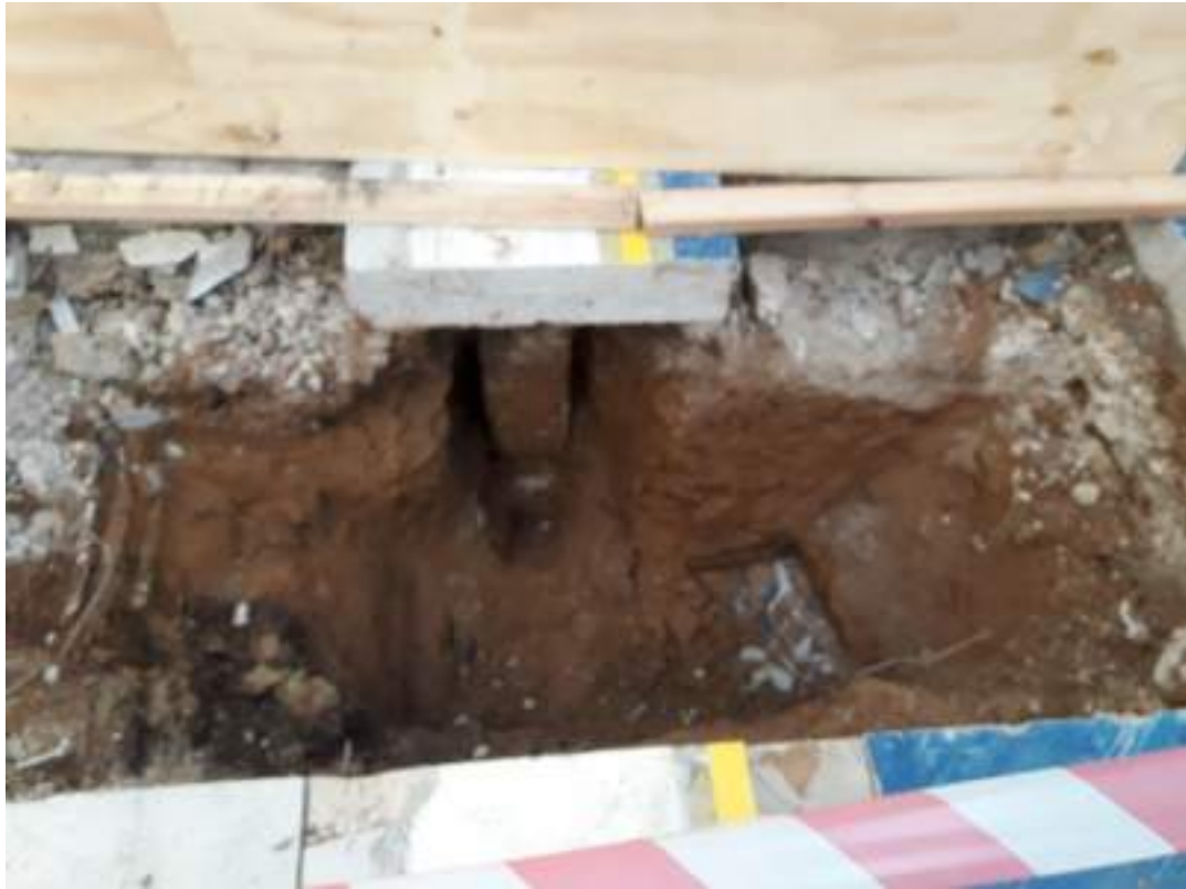
Photo 3: Image of TP03. Note the pile underlying the steel beam 0.20m wide. Base of pile unknown.
