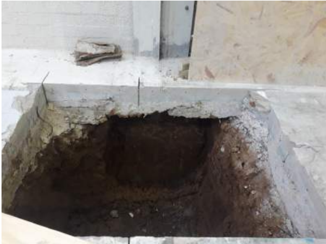
Photo 1: Image of TP01. Note the pile underlying the steel 0.70m wide. Base of pile unknown.
