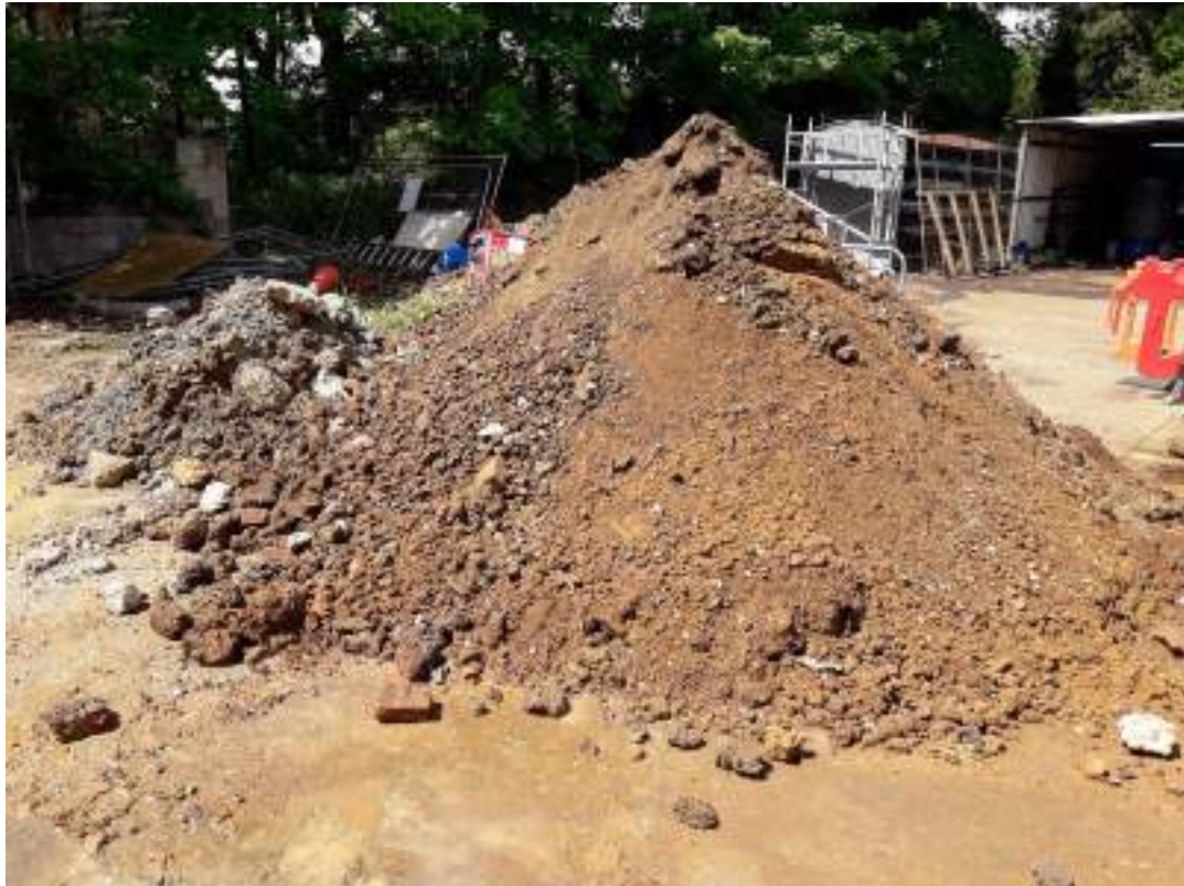
Photo 15: Image of stockpile of material.
