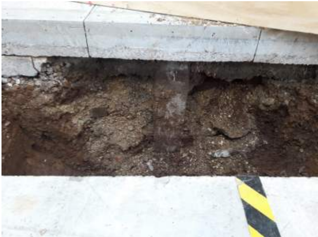
Photo 2: Image of TP02. Note the pile underlying the steel beam 0.20m wide. Base of pile unknown.
