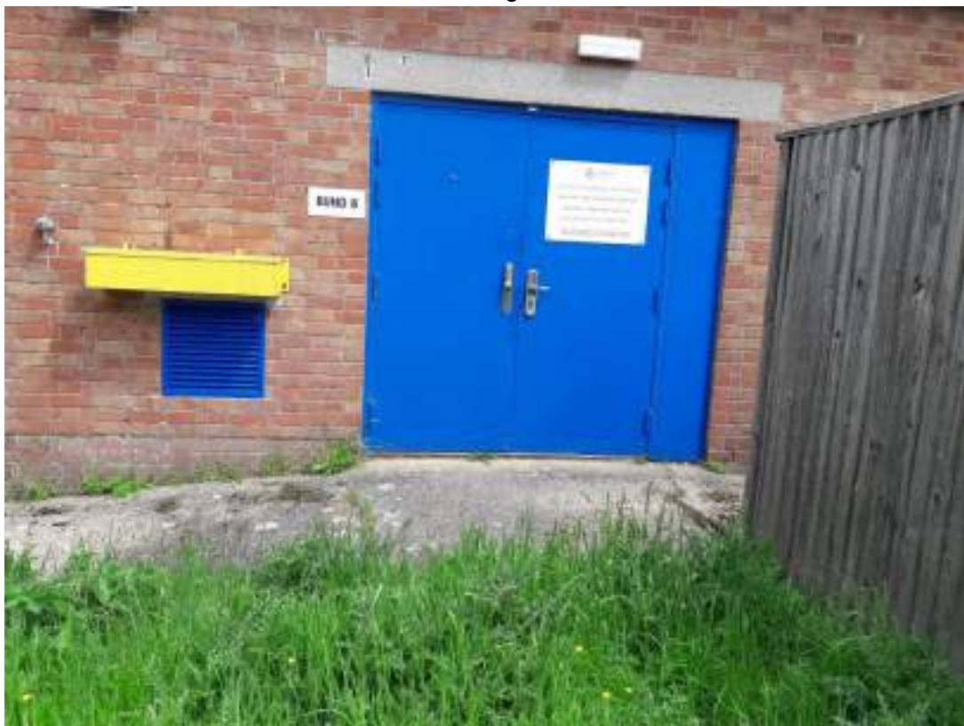
Photo 4: Image of building associated with sprinkler system located north of Site.
