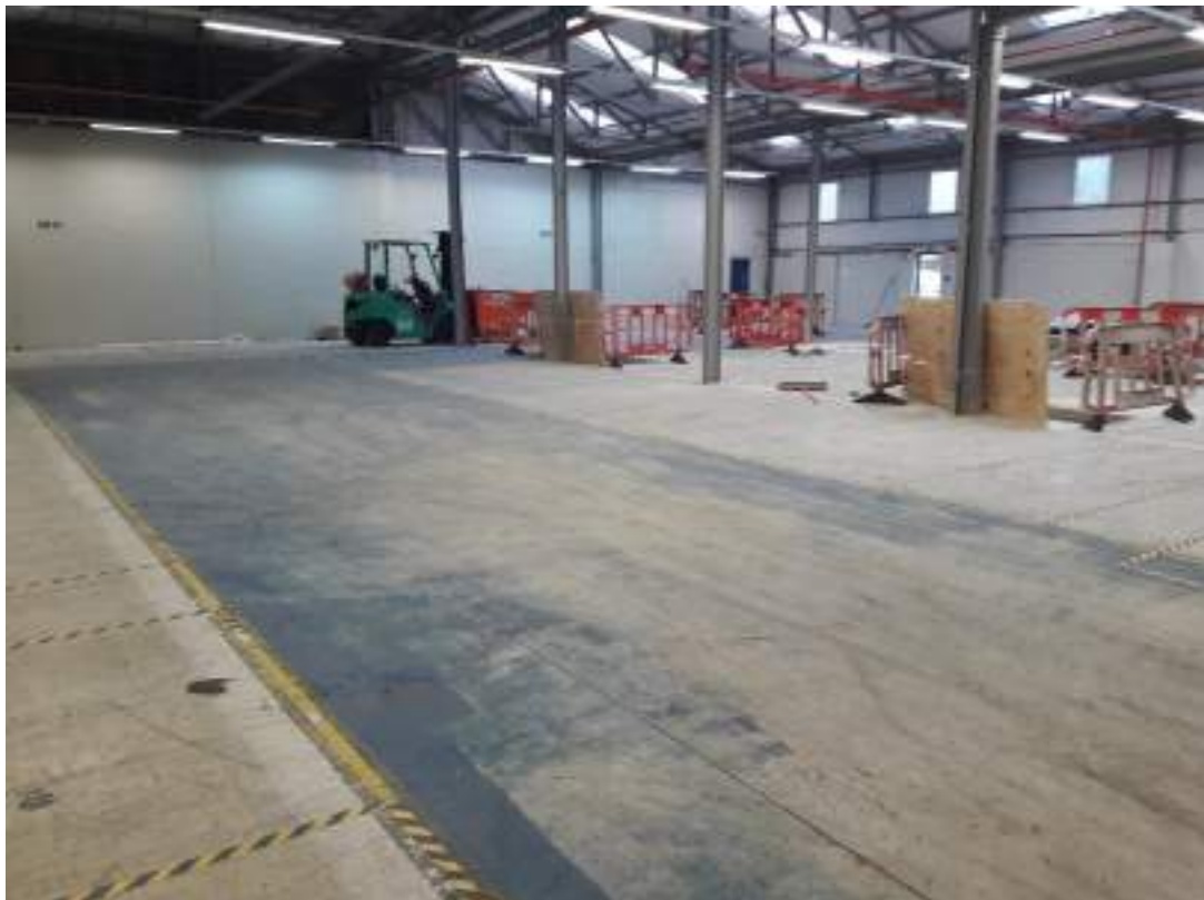
Photo 2: Image of internal commercial building.
