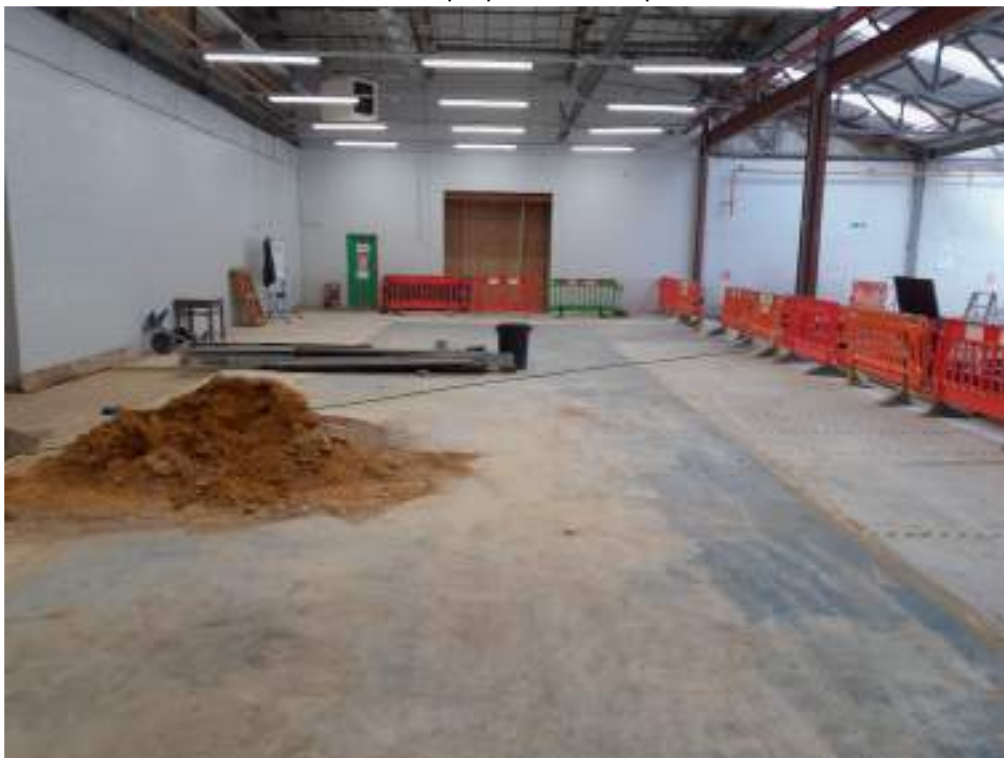
Photo 2. View of the installed concrete base slab looking towards the south-east boundary of the development.
