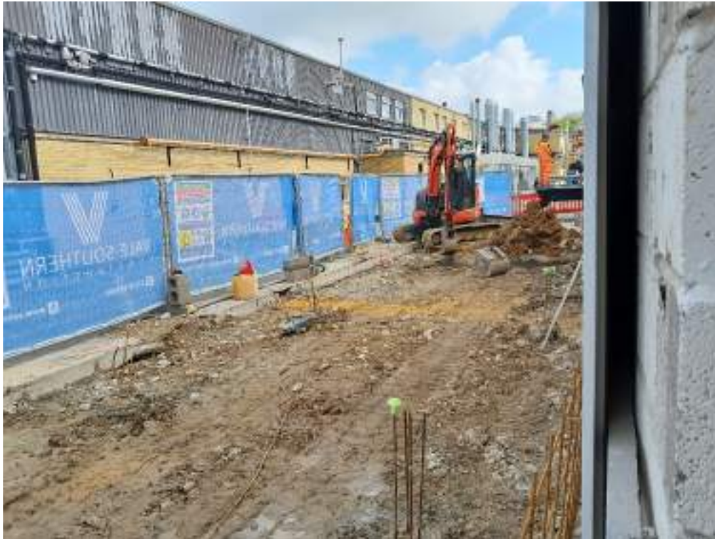
Photo 3. View of the incomplete external area of the proposed development looking north-east.
