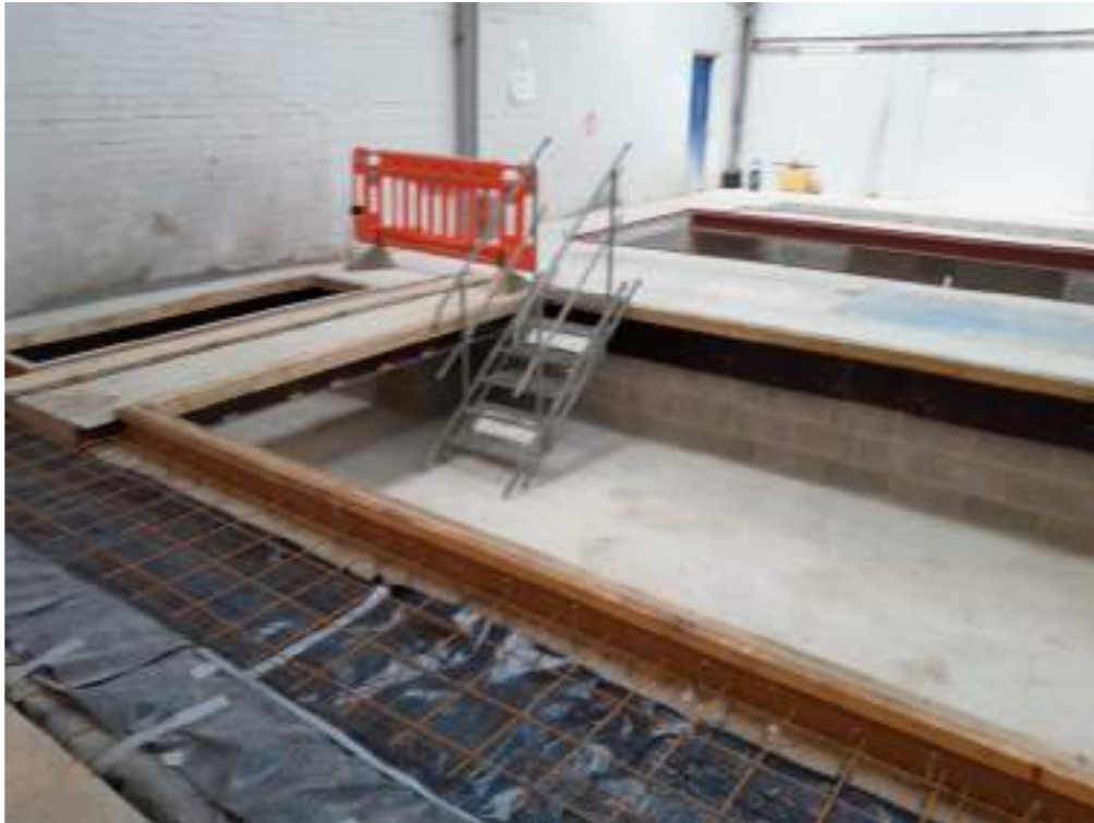
Photo 1. View of the installed concrete ground slab within the interior of the building looking towards the south-west corner of the proposed development.
