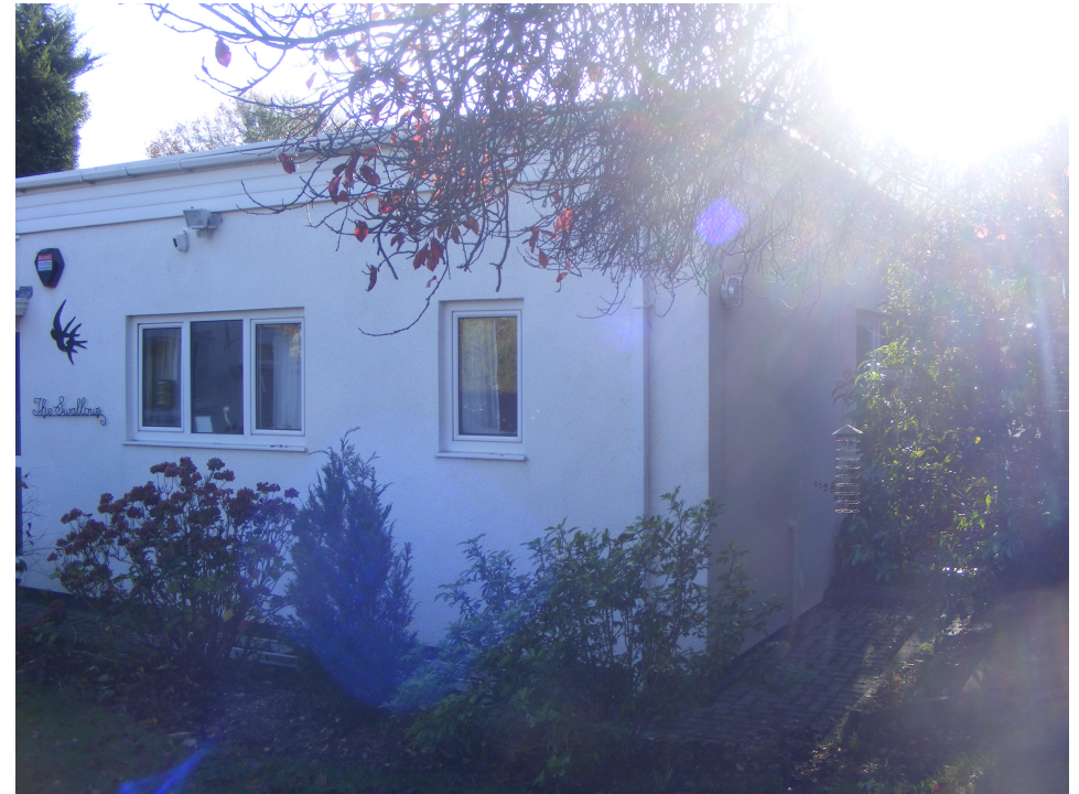
(09) Photo looking South-East at the side of the Bungalow’s Western wing, highlighting the general form and material character for this part of the property.
