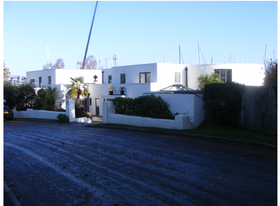
(15) Photo of No.27 Crowsport Estate, a recently extended and remodelled white rendered property with First Floor and Roof Terrace accommodation, as per Planning Approval C/11/69820 (details confirmed in Appendix A).
