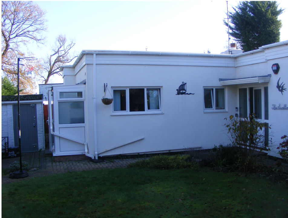
(06) Photo looking East from within the front “Courtyard Style Garden”, highlighting the form, material finish and simple character incorporated into the existing Bungalow’s composition.
