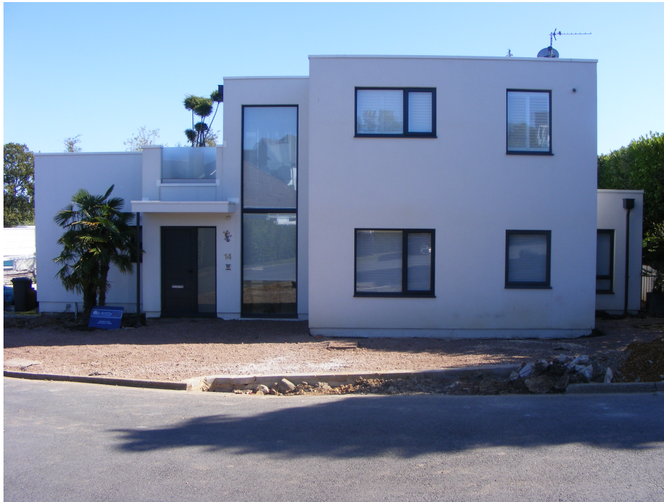
(12) Photo of No.14 Crowsport Estate, recently extended and remodelled to include new first floor accommodation and an associated roof terrace, as per Planning Approval C/15/76351 (details confirmed in Appendix A).
