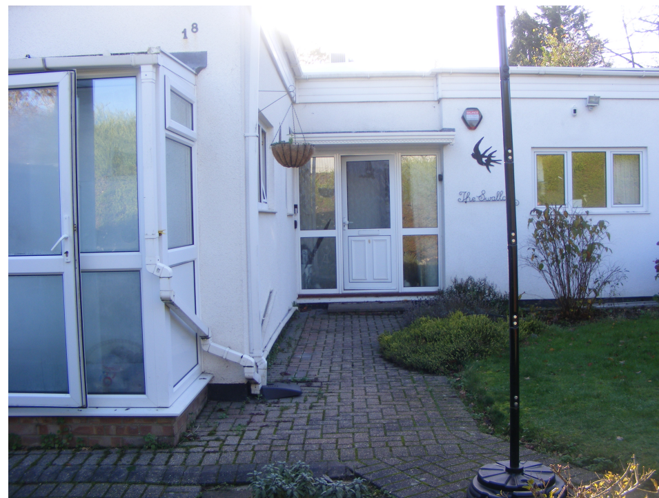
(05) Photo looking south from within that site at the Bungalow's existing front door and block paved approach, highlighting its white rendered material finish, with simple window opening character.
