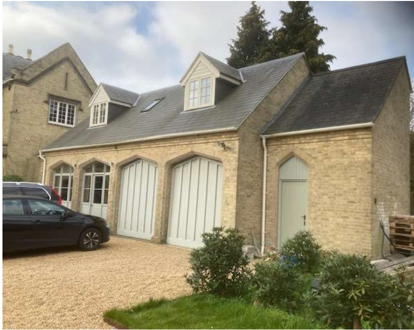
Fig.2 – Photograph showing the garage extension at Hoe Moor House.
