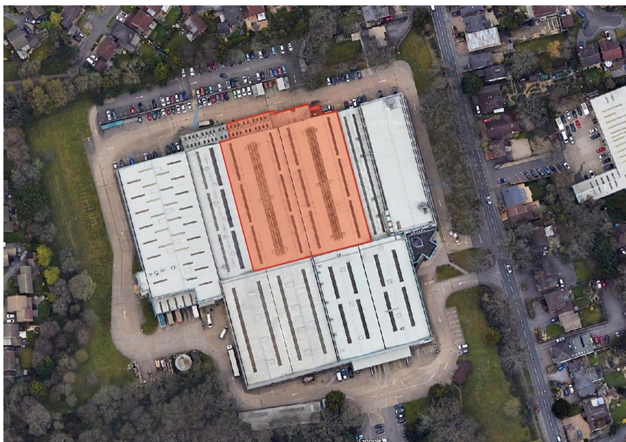
Aerial photograph showing the area of the building affected edged and colour washed in red © Google Maps 2023
