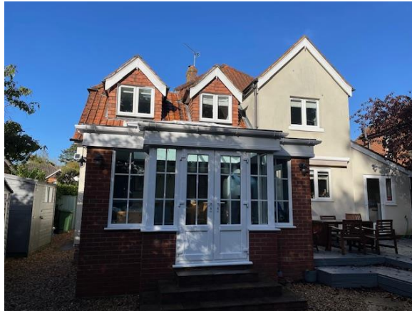
Photo 2: Rear elevation of house.
