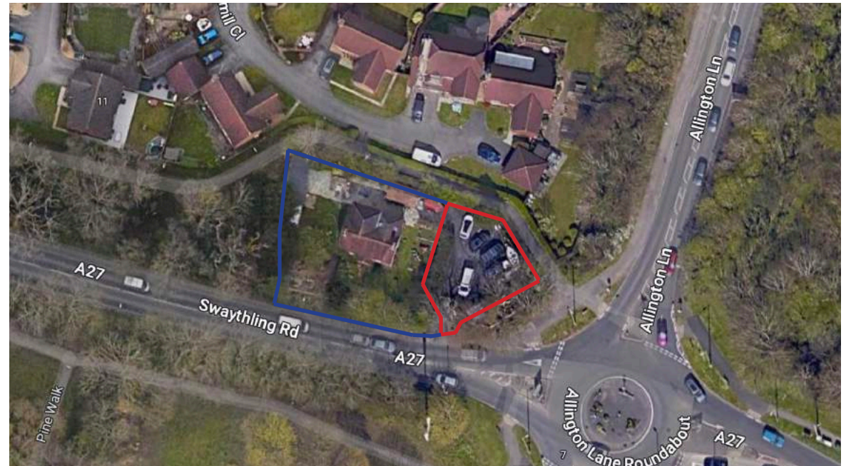
Fig. 1 | Aerial View of site
