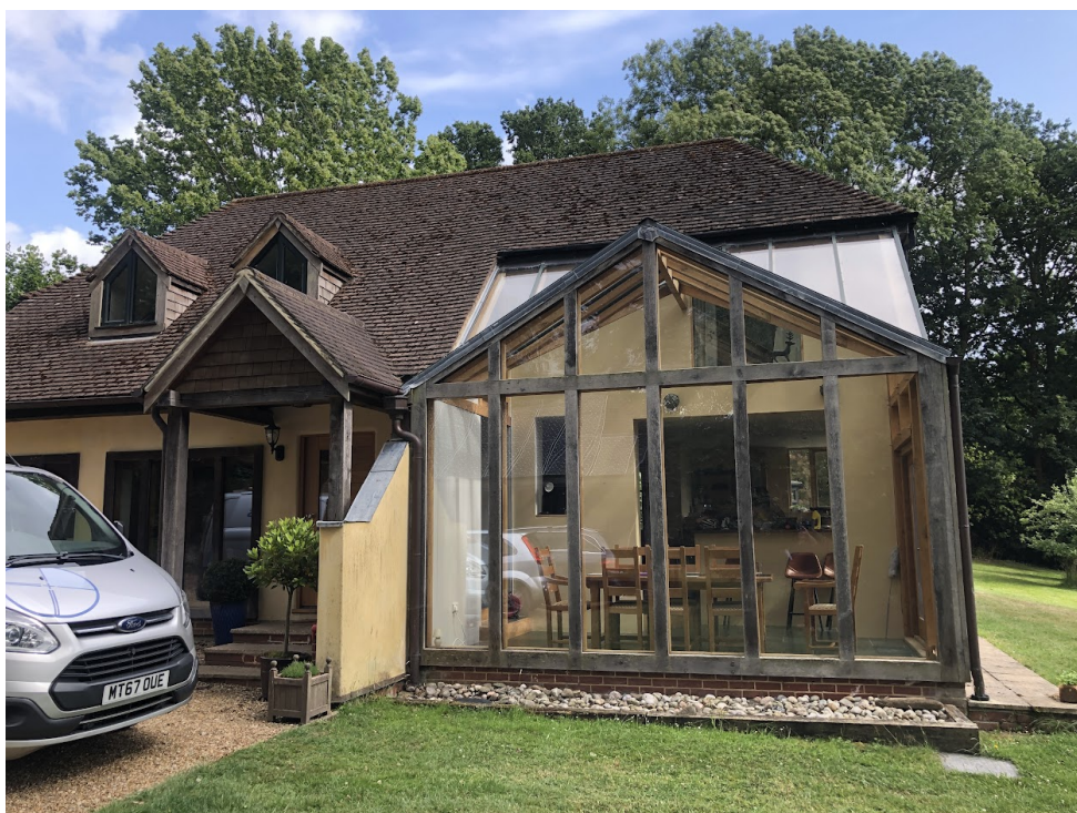
Photo 1: Front north elevation.
