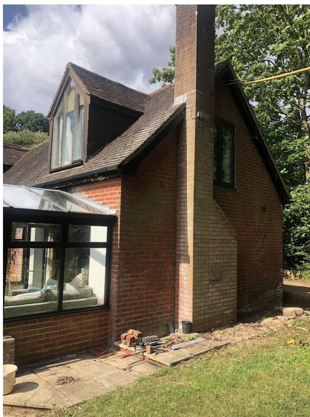
Photo 5: South elevation of south wing gable end
