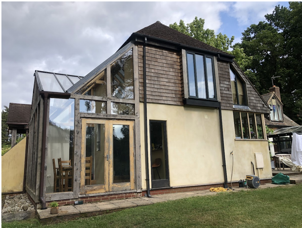
Photo 7: West elevation of north wing
