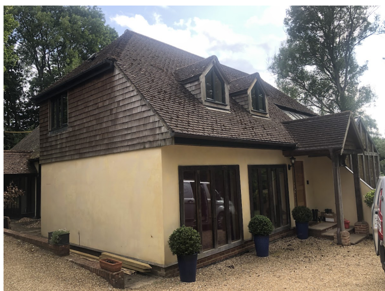
Photo 2: North and part east elevation
