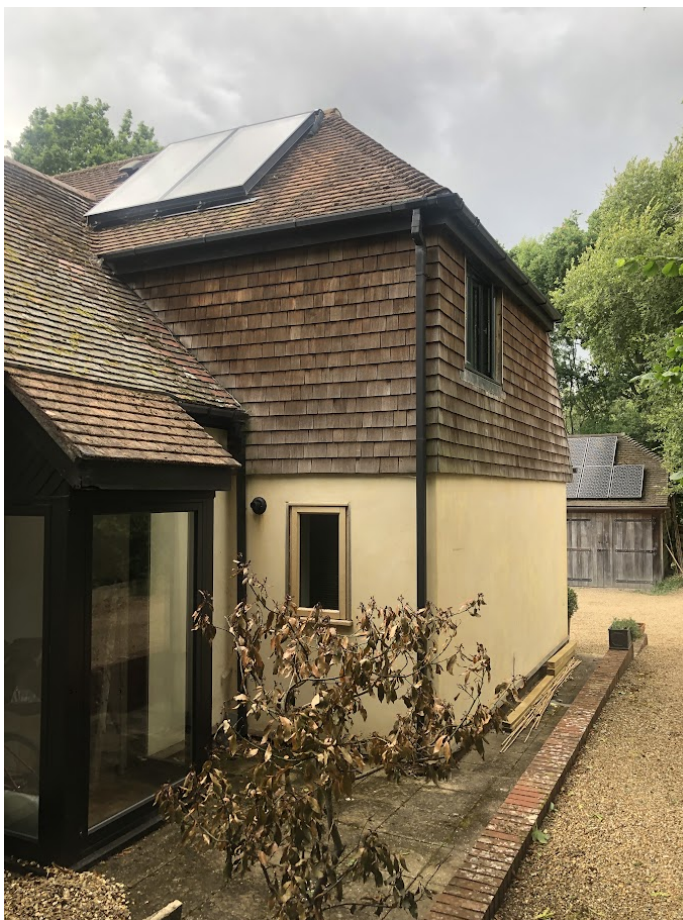
Photo 3: East elevation of north wing
