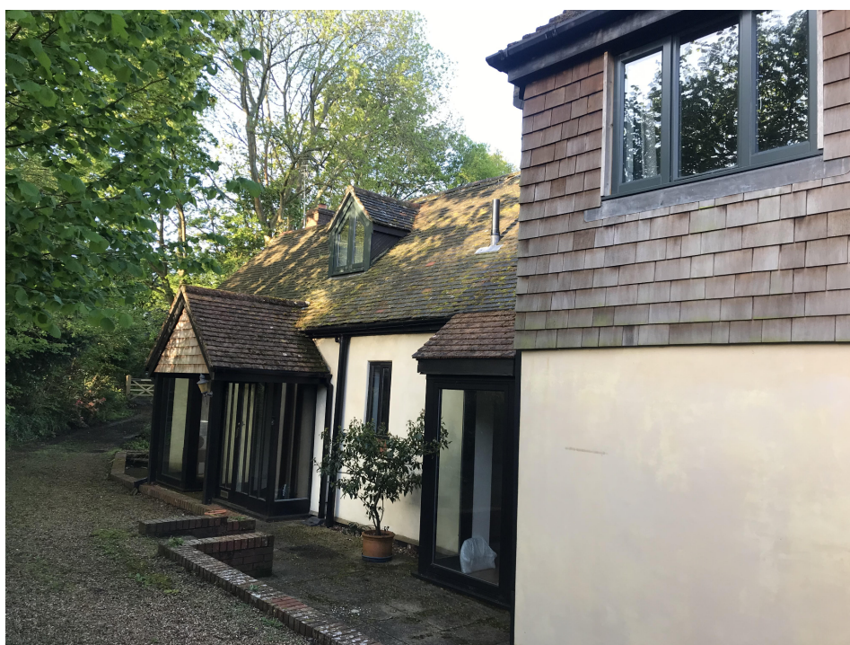
Photo 4: East elevation of south wing
