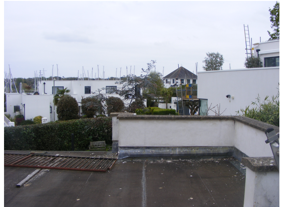
(13) Roof Top Photo (C) looking South-East from the existing Roof Level on No.20, seeking to highlight general views available and the minimal impact on any surrounding properties.
