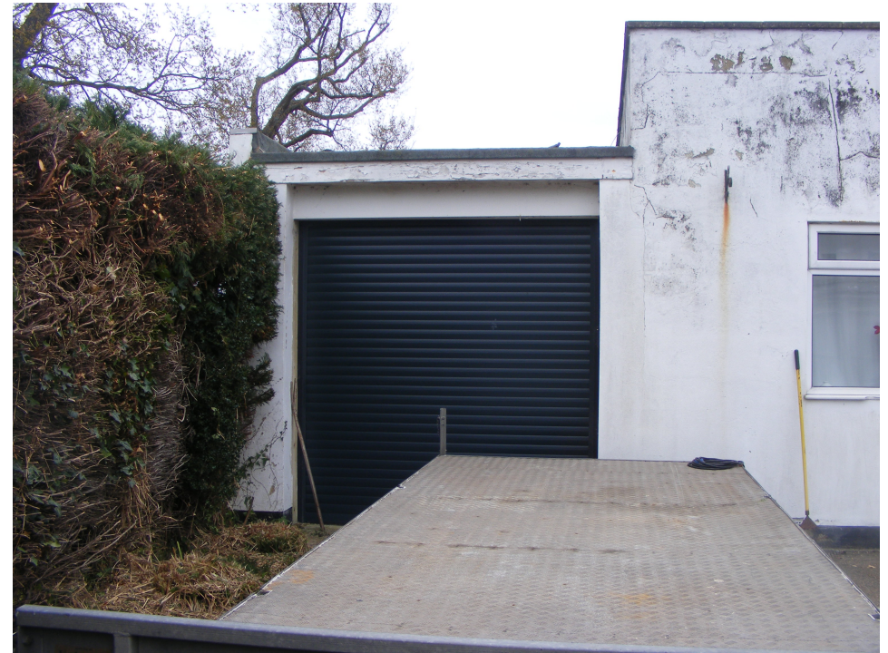
(03) Photo looking East at the front of the existing attached Garage, due to have the roof raised and provided with new parapet walls and coping above.
