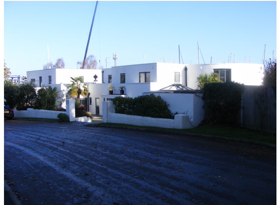
(15) Photo of No.27 Crowsport Estate (opposite No.20), a recently extended and remodelled white rendered property with First Floor and Roof Terrace accommodation, as per Planning Approval C/11/69820 (details confirmed in Appendix A).
