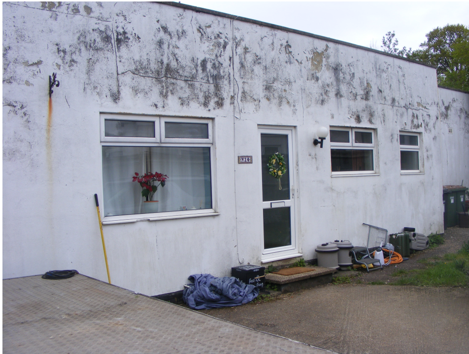
(02) Photo looking South at No.20's front elevation, highlighting its material character, the proportions of the existing window and door openings, and the weathered condition of the elevation.
