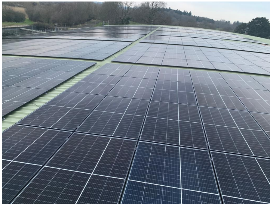
Image showing similar arrangement at PW Itchen site
