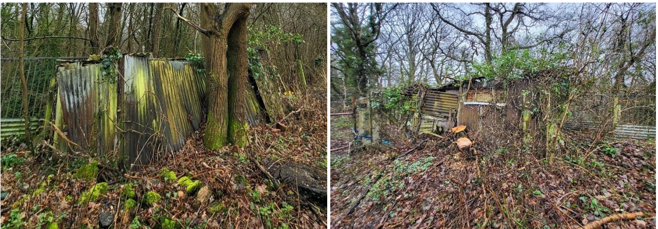
Figure 13. View of the sheds on site
