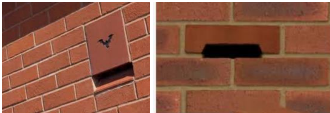
Figure 28. Example of bat bricks in external walls
