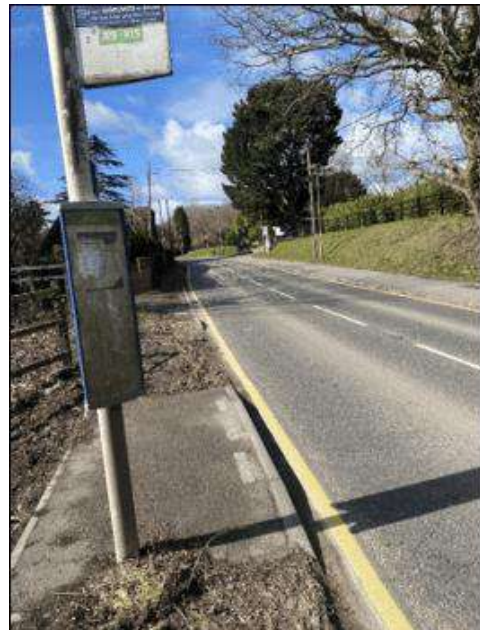
Photograph 5: Existing Conditions Westbound
