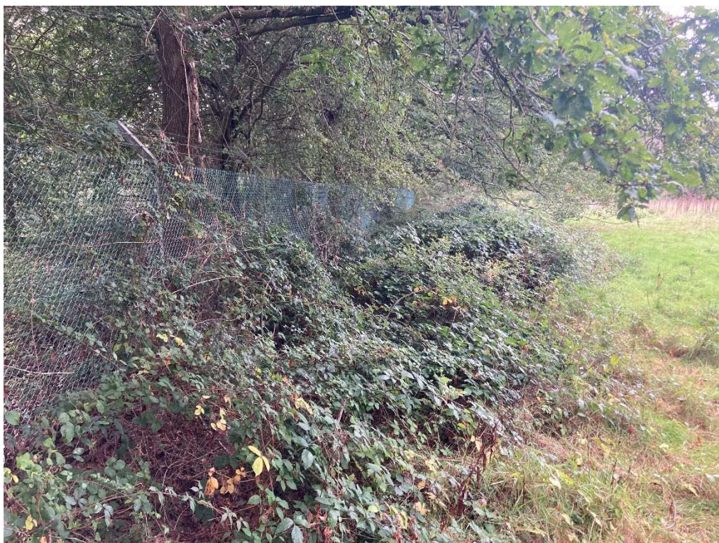
Photograph 6: Metal post and mesh fence along southern boundary, adjacent to railway cutting.
