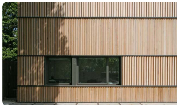
High quality vertical timber cladding (VG Sila cladding, Russwood)
