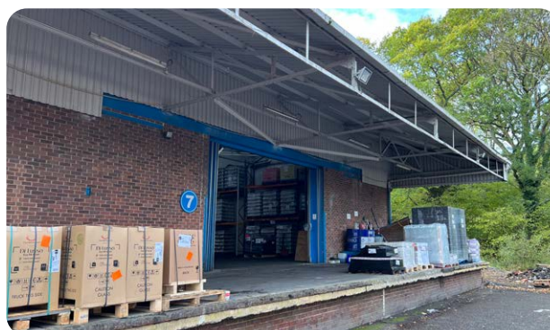
Unit 7 - brickwork & steel structure frame
