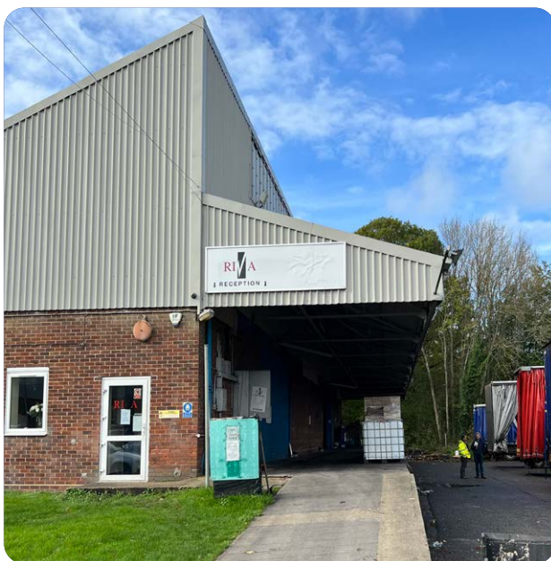
Loading area to existing commercial unit
