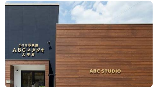
Horizontal timber & dark grey cladding provides a high quality finish
