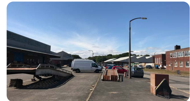
The central estate road access to Chalcroft Business Park
