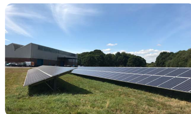
Solar panel field, building 9 in background
