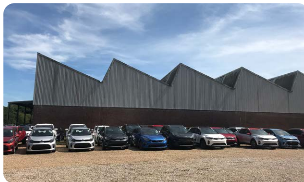
Building 9 South-East elevation
