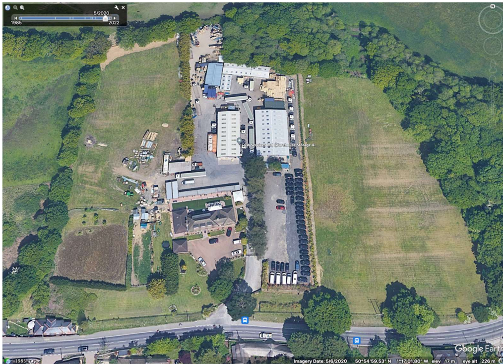
Aerial view taken on 6 th May 2020.
