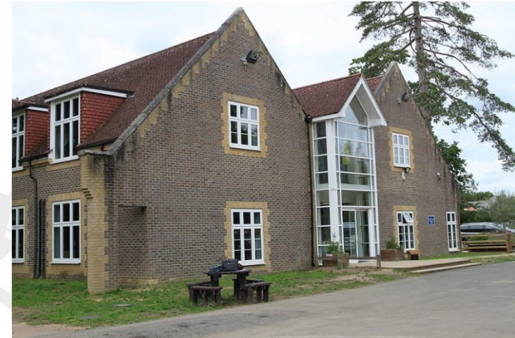
Photograph 1 – main entrance to the Main School building (north-east elevation)
