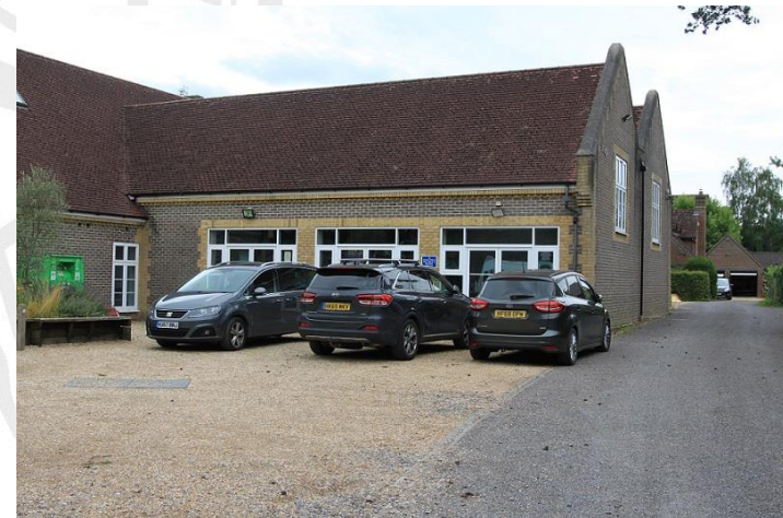
Photograph 2 – the school hall on the north-west side of the Main building
