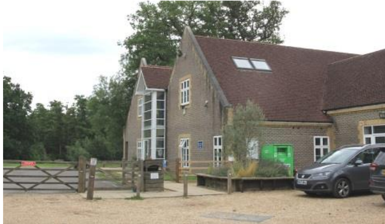
Photograph 7 – north-east elevation of Main School building
