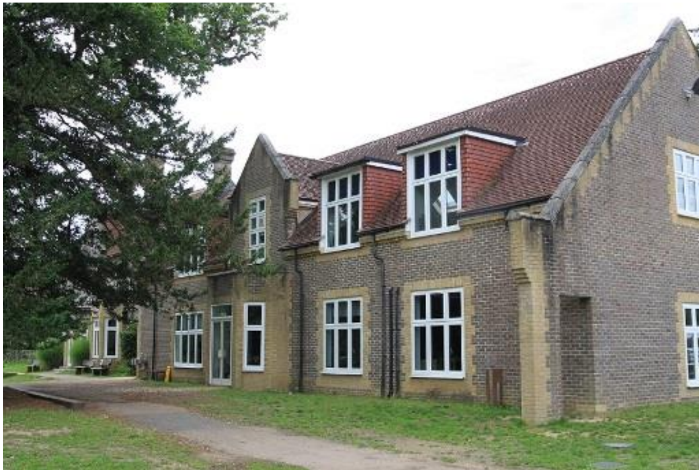
Photograph 6 – the terrace in front of the south-east elevation of the Main School building
