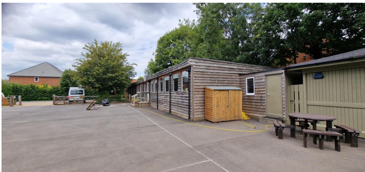
Picture 2: Building A will be removed during the works
