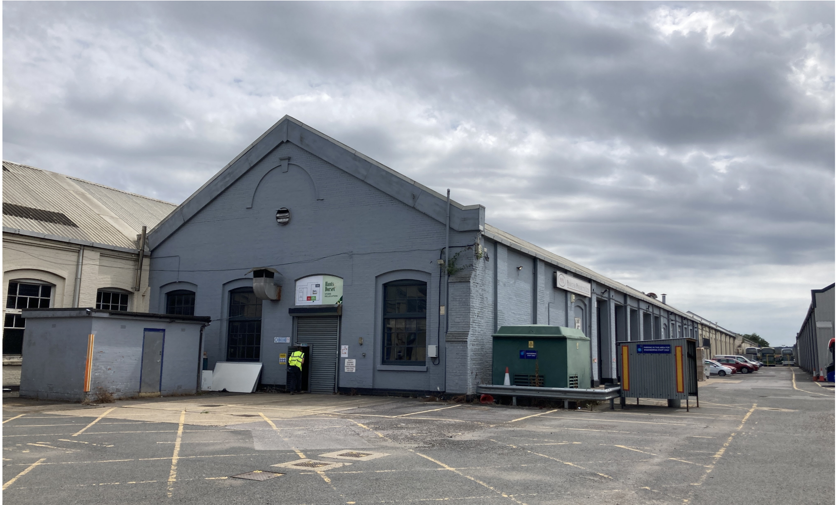
Figure 3 Existing (internal) North Elevation
