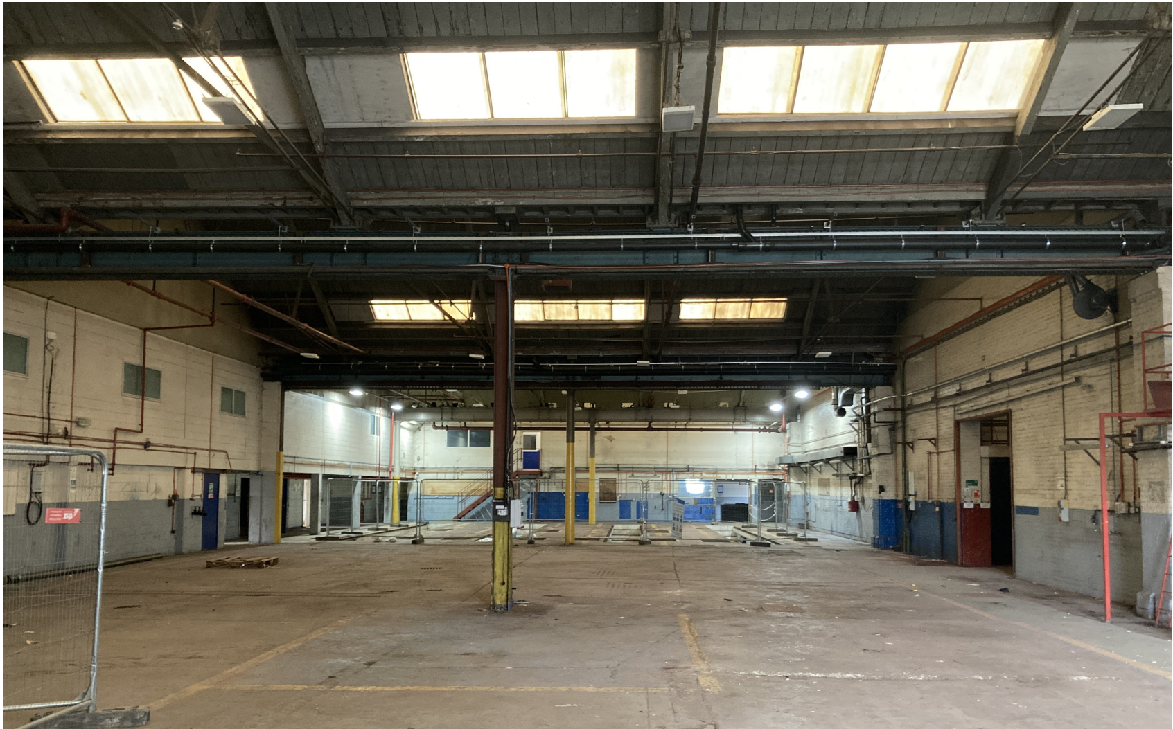
Figure 5 Existing Internal view from the western roller shutter door
