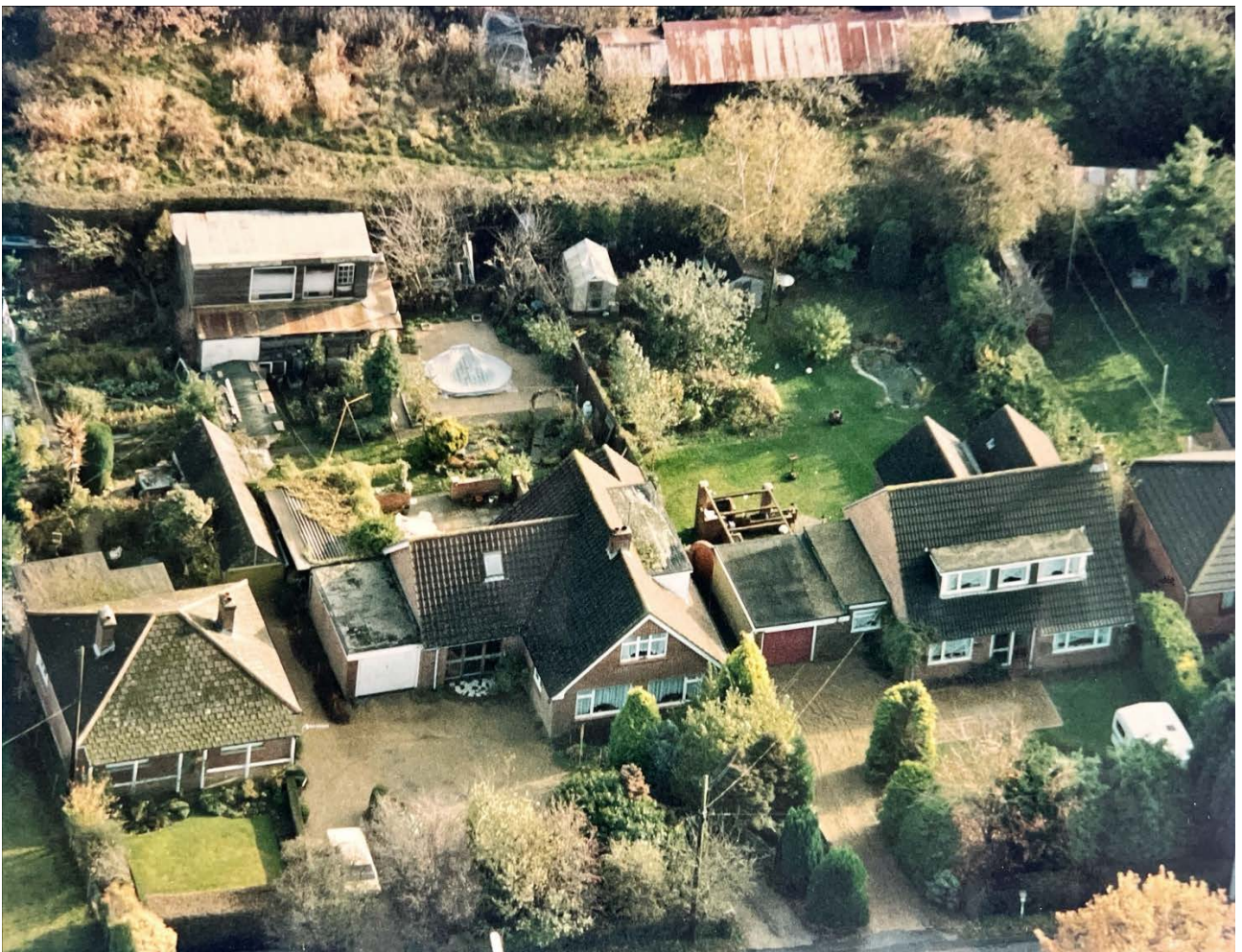
Fig 1. Aerial view prior to removal of two storey workshop and lean to.
