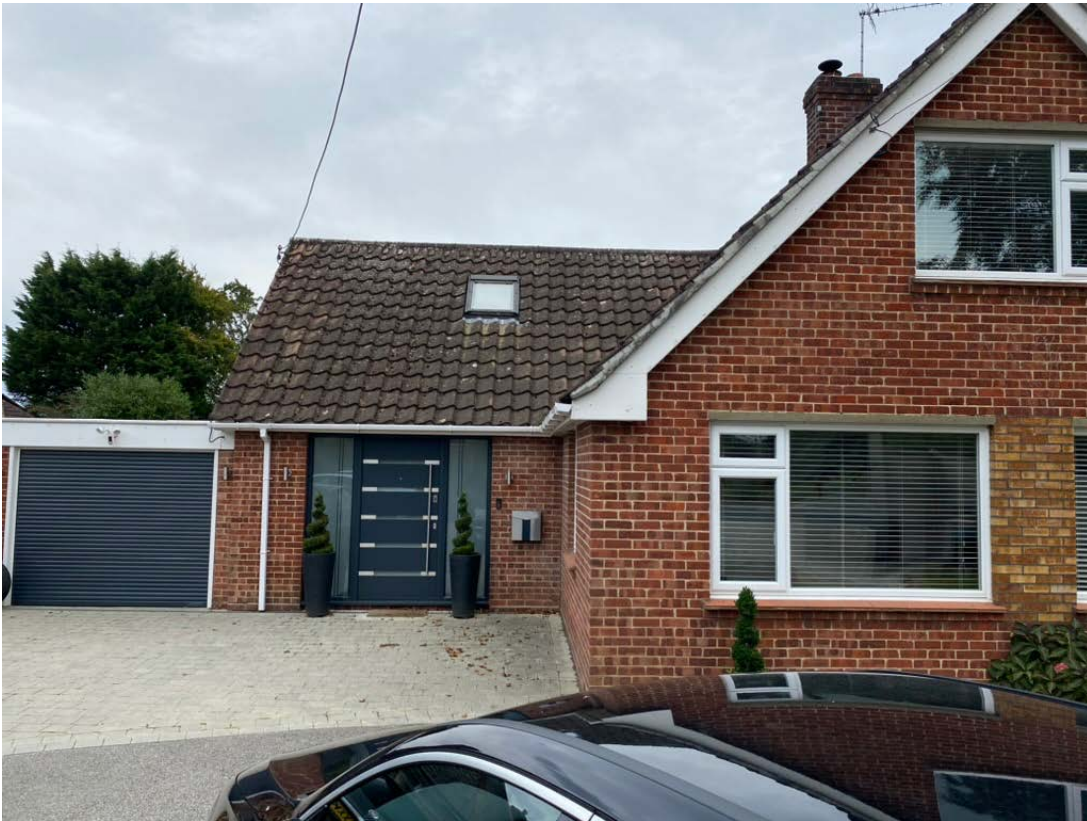
Fig 2. View of Front Elevation.
