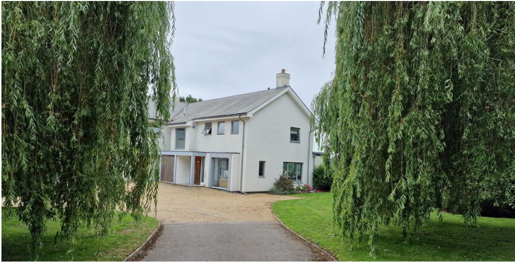
View of the existing house from entrance to the site off High Street
