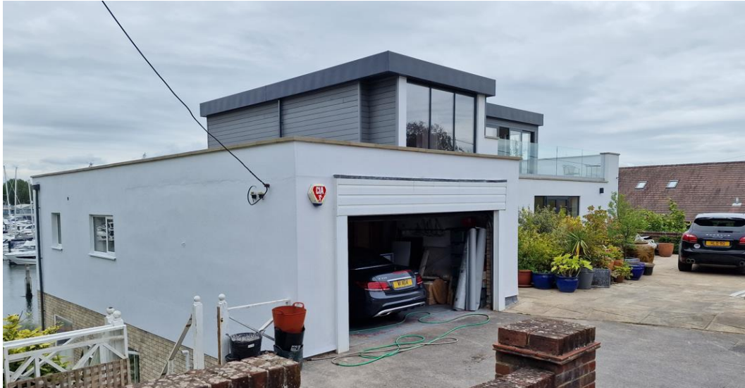
Side and front elevation to the recently remodelled and extended dwelling known as Waters Edge, Lands End Road
