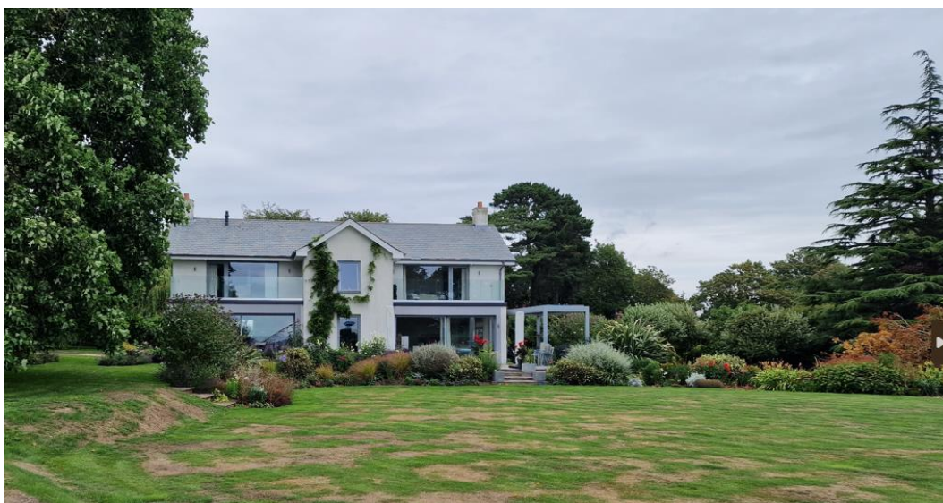
Existing rear elevation of the dwelling
