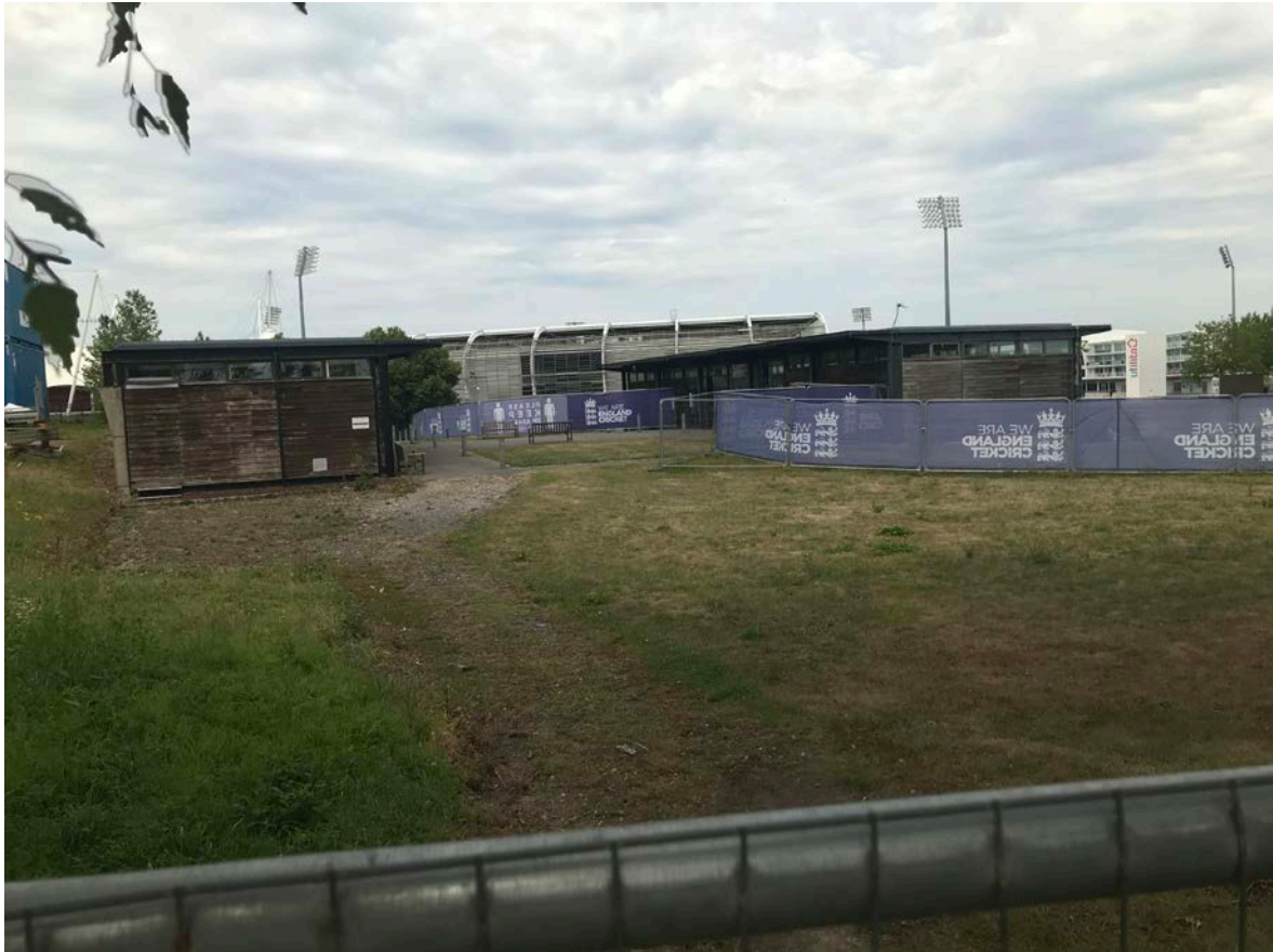
Plate 5: 2020 view facing north of existing golf club buildings to the south of the Ageas Bowl and within the area of indicative development to the south of the stadium
