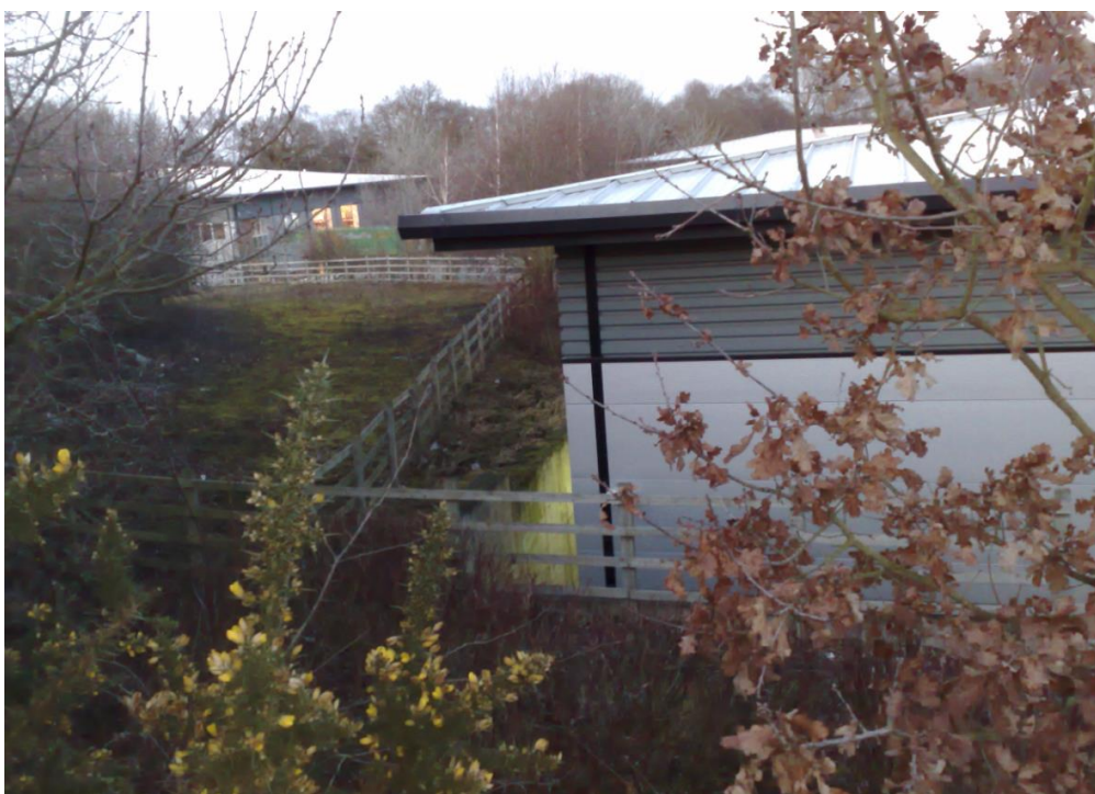
The Southwest corner of Unit 5
