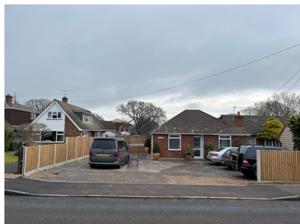
The site viewed from the west, on Botley Road.
