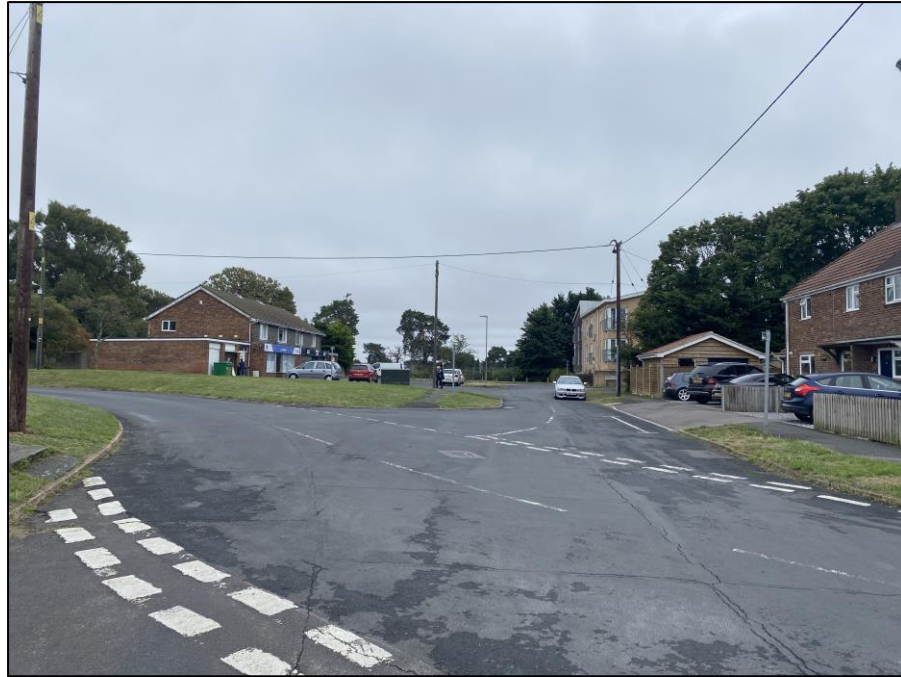
Photograph 2: Existing Access (Castle Road / Queens View Junction)
