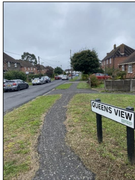
Photograph 5: Queens View Footways
