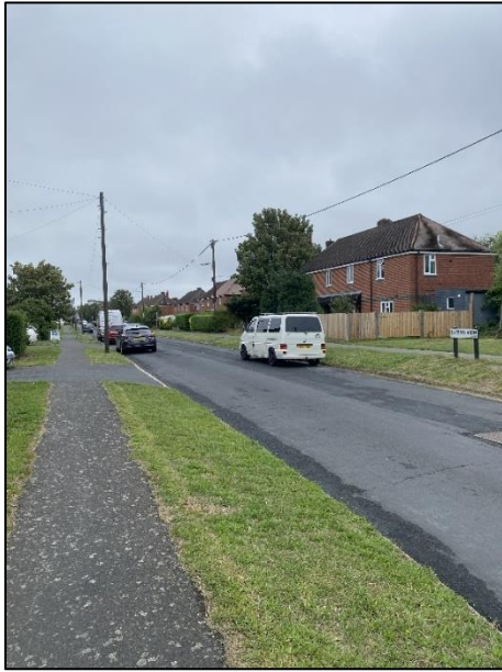
Photograph 4: Queens View Footways
