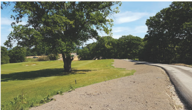
2. View looking east along the existing road/track
