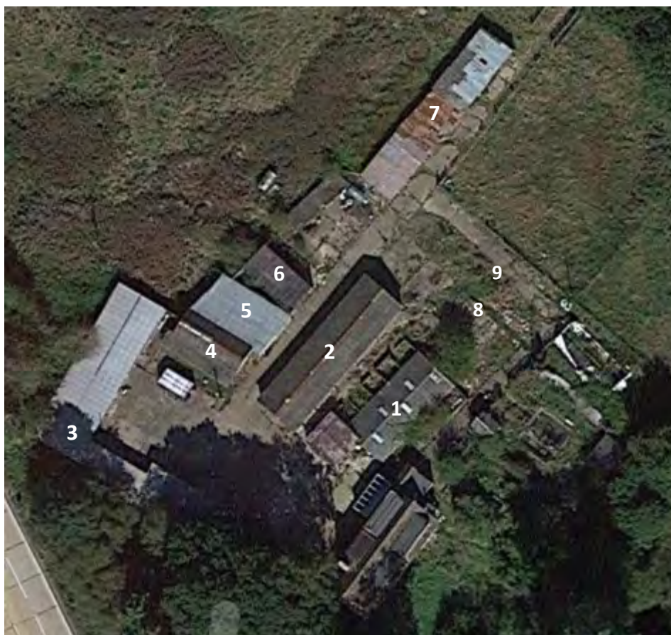
Figure 14. The 9 outbuildings on site with their associated numbers.
