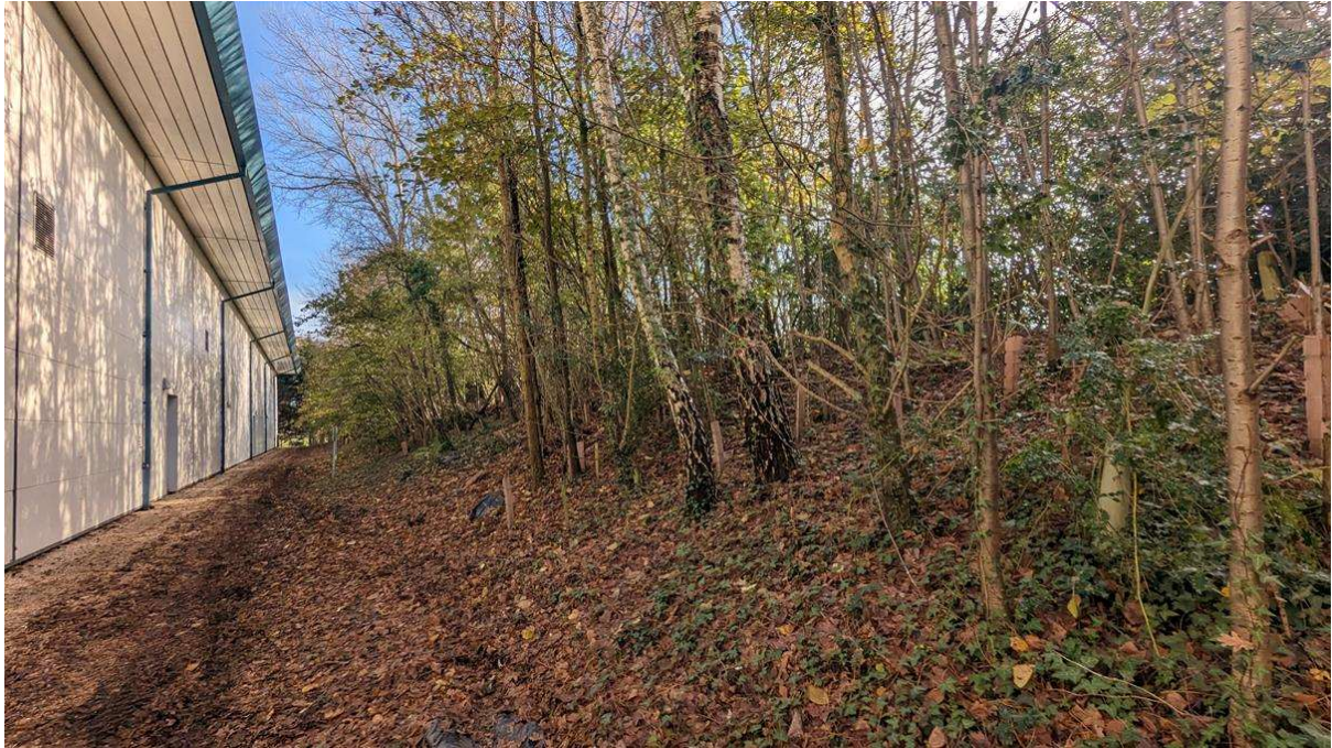
Photo 7 – View of the rear (south) of the building with gravel and woodland.
