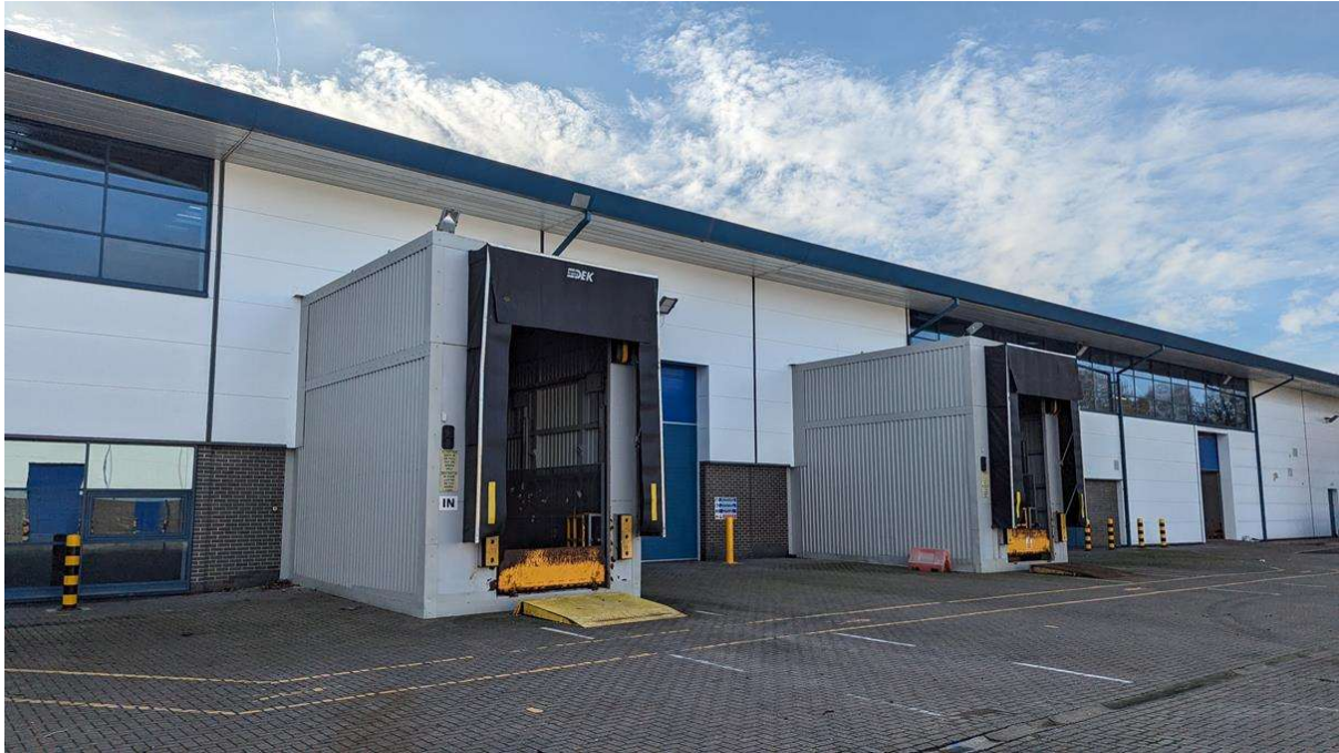
Photo 3 – View of the loading bays.
