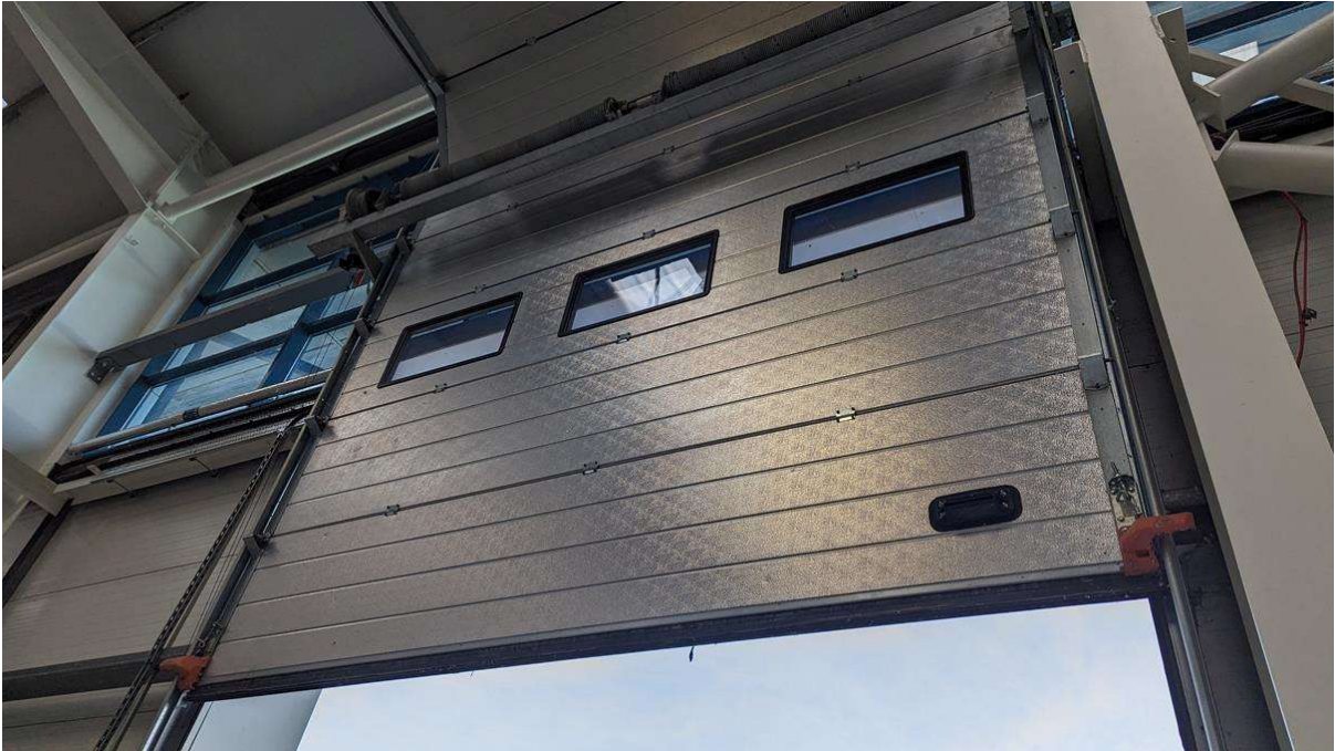
Photo 5 – View inside the roller-shutter doors.
