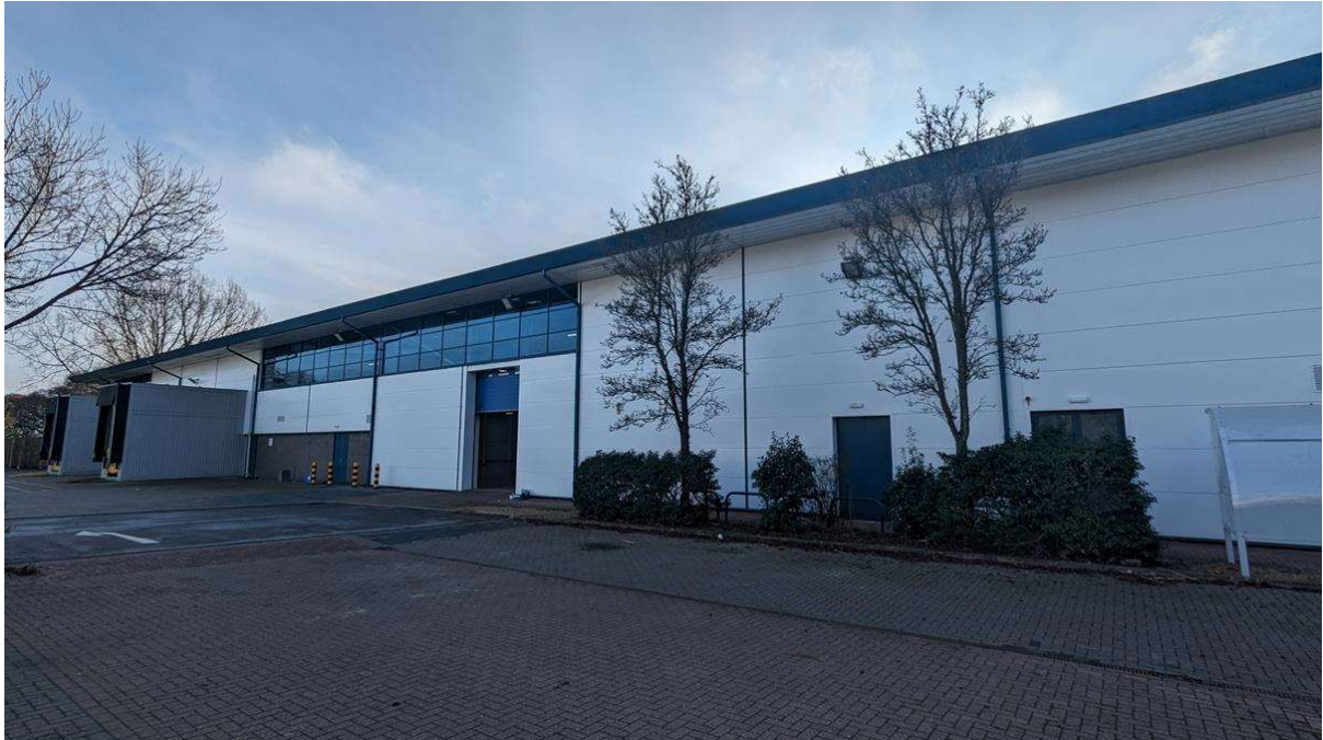
Photo 1 – View of B1 from the north. Note loading bays.
