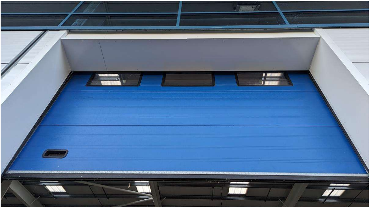
Photo 6 – External view of the roller-shutter doors.
