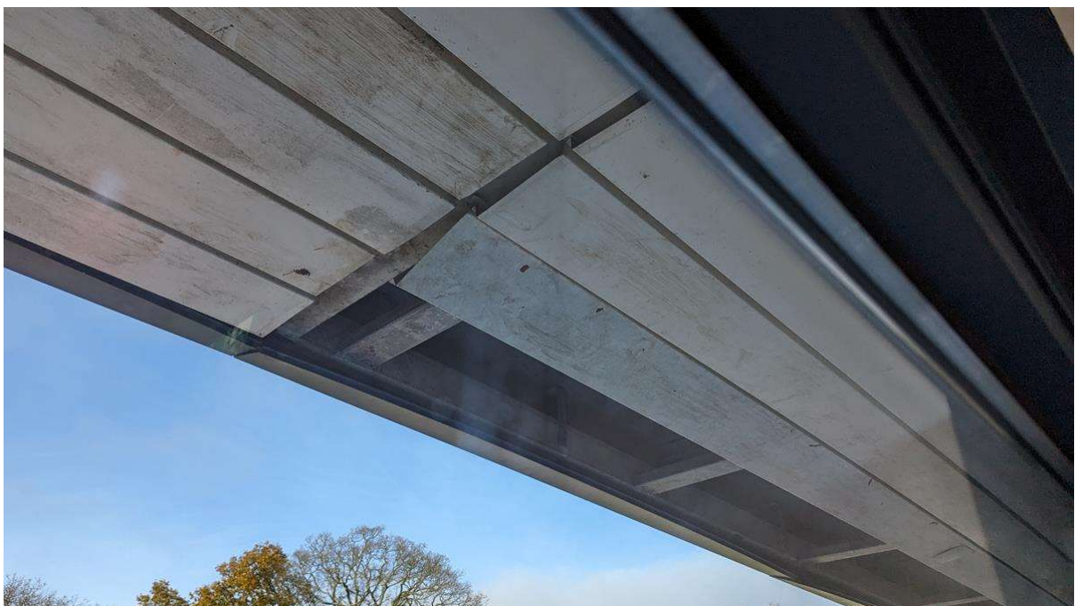
Photo 2 – Limited view inside the soffit from the top floor.
