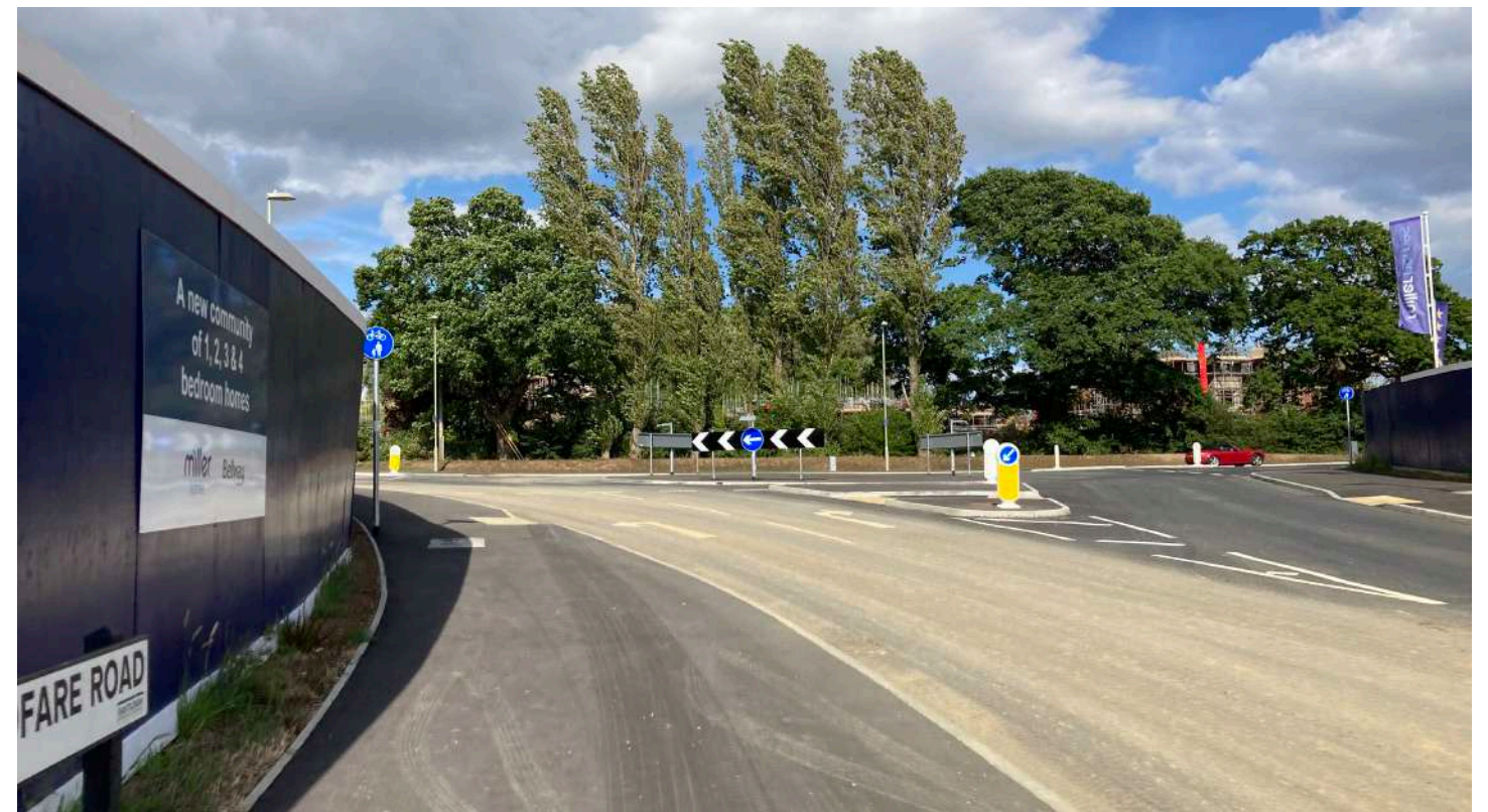
View of new roundabout junction between Fieldfare Road and Winchester Road
