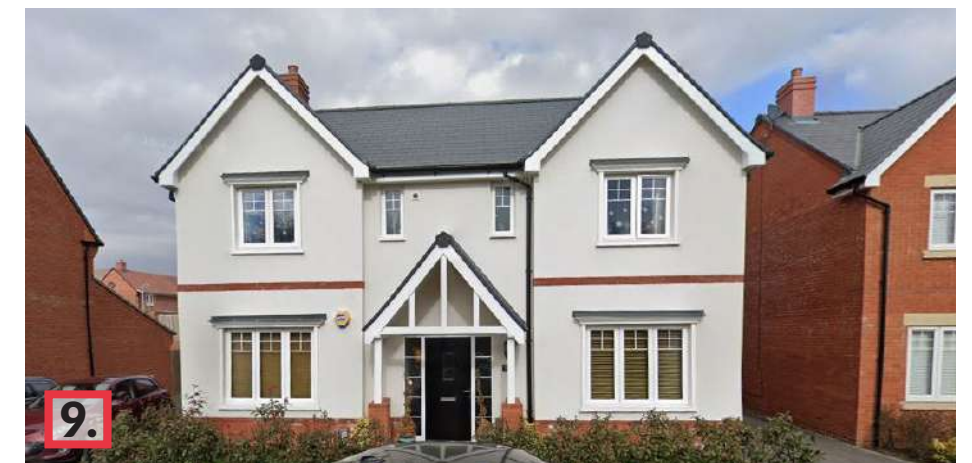
Braxells Road - Residential Dwelling
