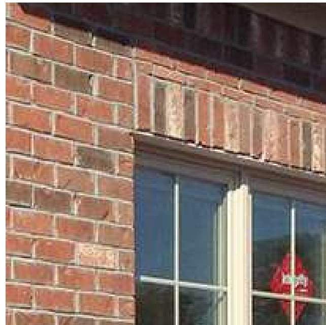
Brickwork window head
