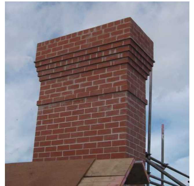
Corbelled Brickwork Chimney Stacks
