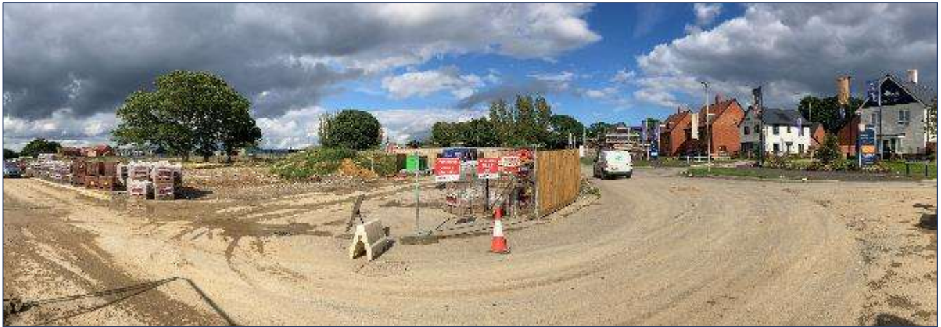
Figure 2.1: View northwards across the site (July 2023) - Bellway sales area to the right of view
