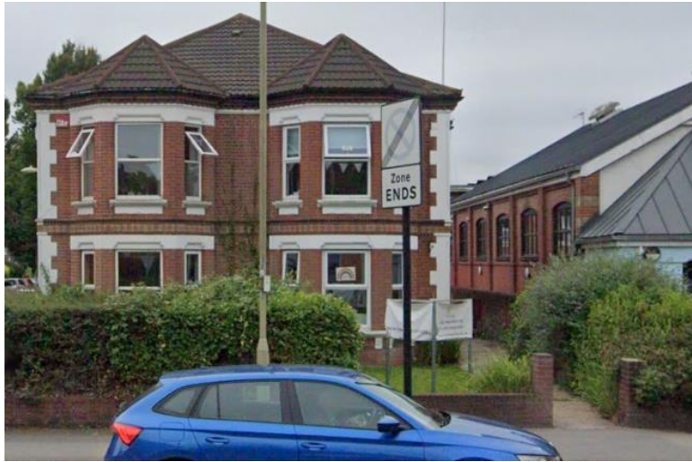
Photo of No 75 and 77 showing the existing gap in the hedge and low wall
