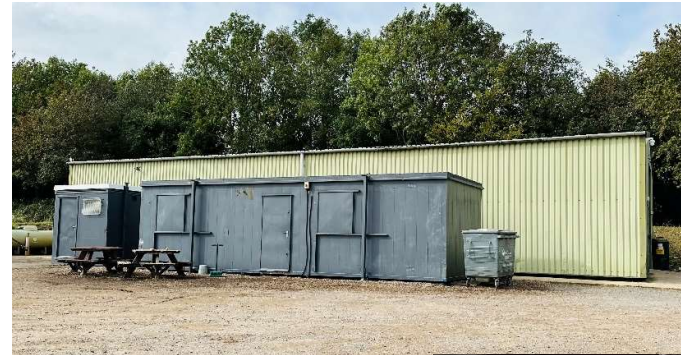
Temporary welfare facilities at the existing Store
