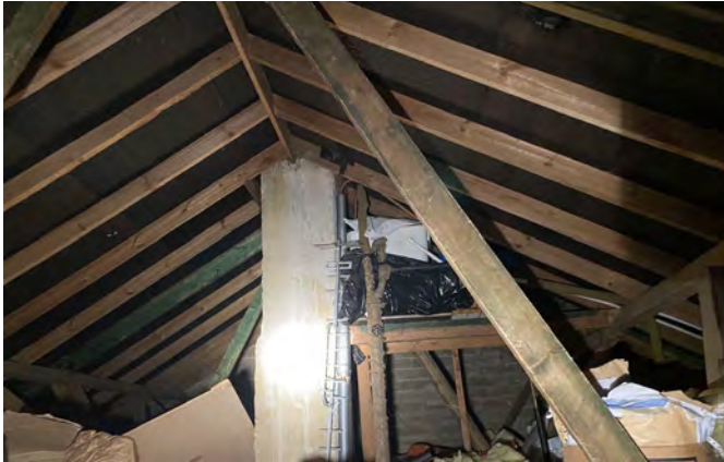
Figure 20. Internal view within the loft space of the dwelling (taken June 2022).
