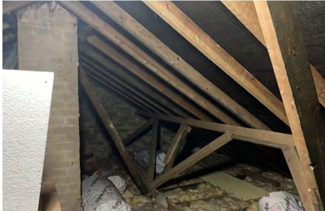
Figure 16. Internal view of the loft space of the dwelling (taken June 2022).
