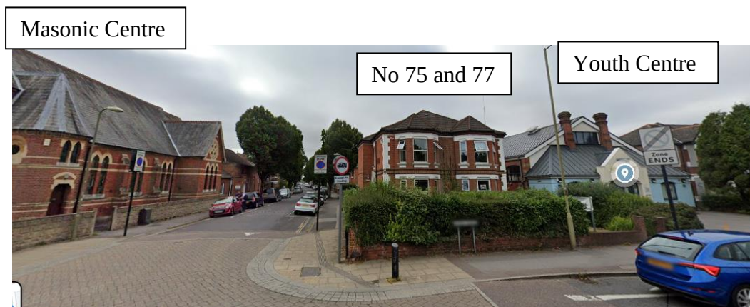
Figure 1 - the location of No 75 and No 77 in relation to its neighbours (courtesy of Google Maps)
