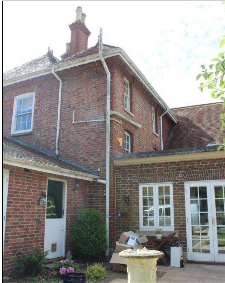
Photograph 10 Narrower, rearward extension to east wing
