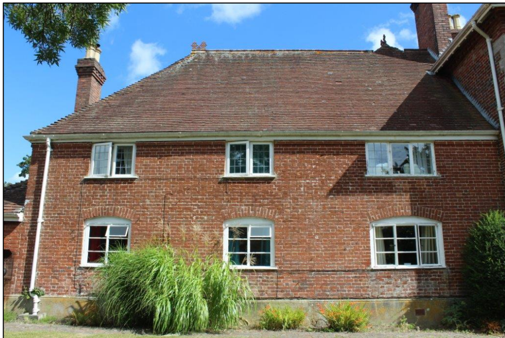
Photograph 12 Principal elevation on south wing
