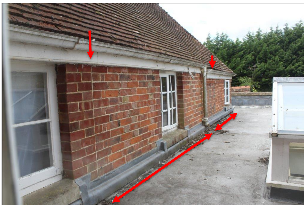
Photograph 13 Rear (north) elevation of south wing
