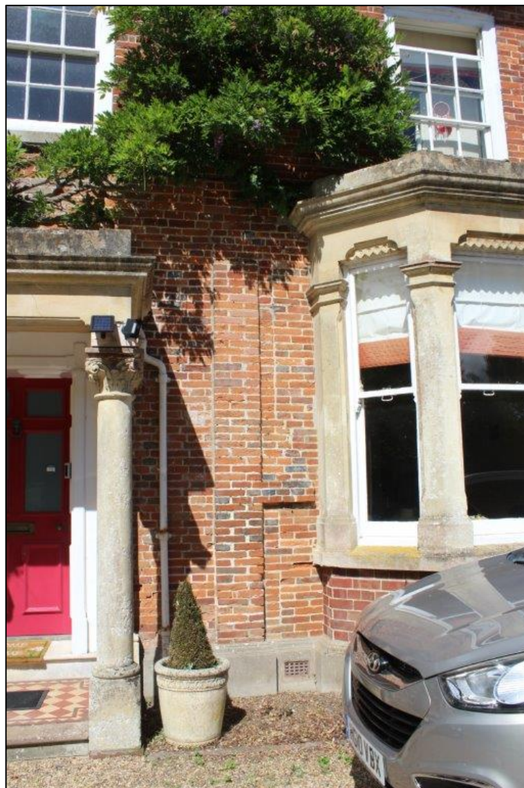
Photograph 8 Detail of east (front) elevation
