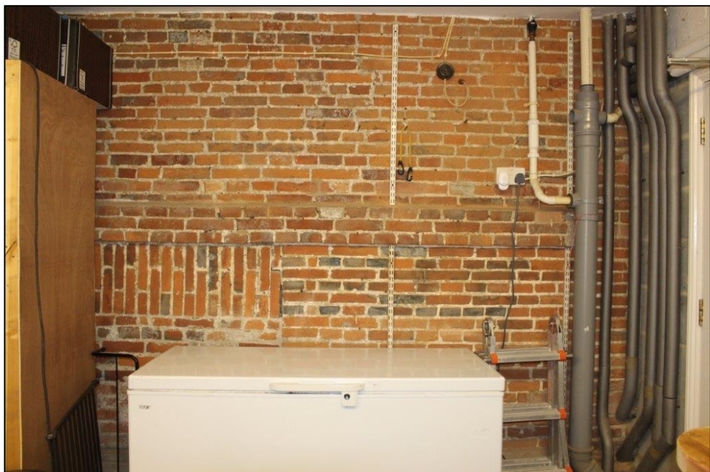
Photograph 11 Narrower, rearward extension to east wing
