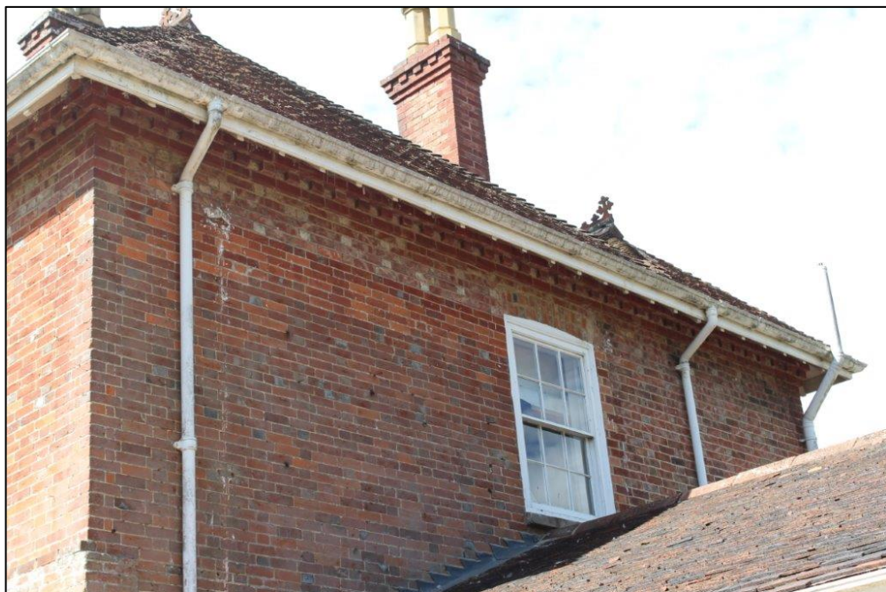
Photograph 9 North elevation of east wing
