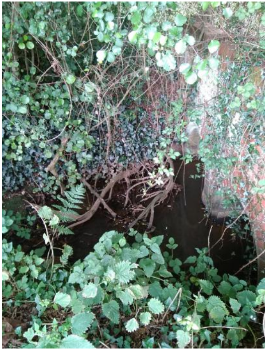
Plate 4: Reach 6. Inflow of southern boundary channel through twin culverts
