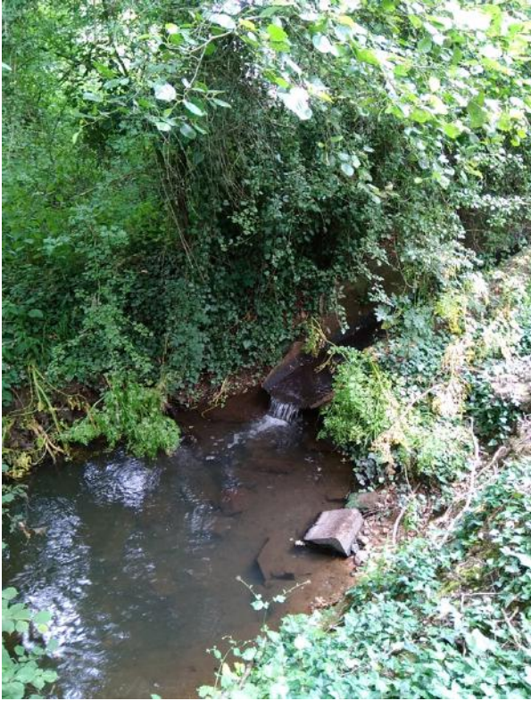
Plate 32: Reach 1. Confluence with Reach 3, barrier to fish migration and artificial (concrete half pipe) channel.
