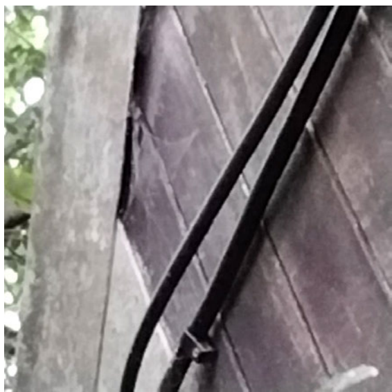
Ref. Sample 22: External. Exterior. Cement roof edging boards
