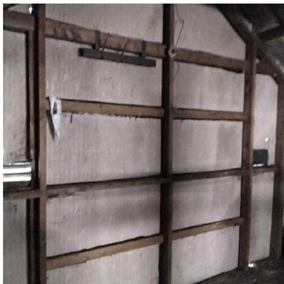
Ref. Sample 22: External. Exterior. Cement roof edging boards
