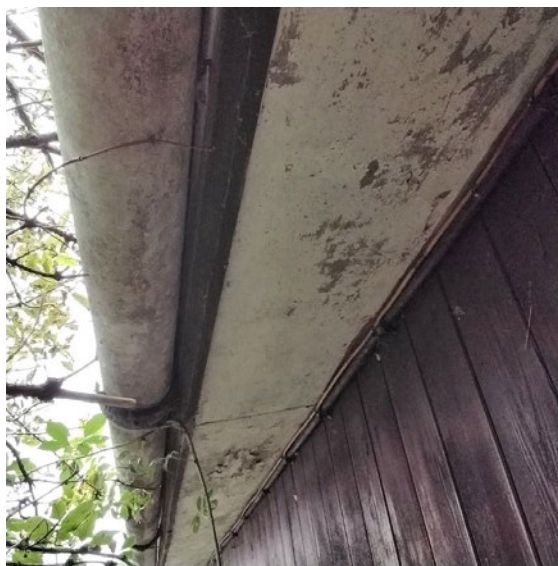
Sample 25: External. Exterior. Cement soffit boards around perimeter
