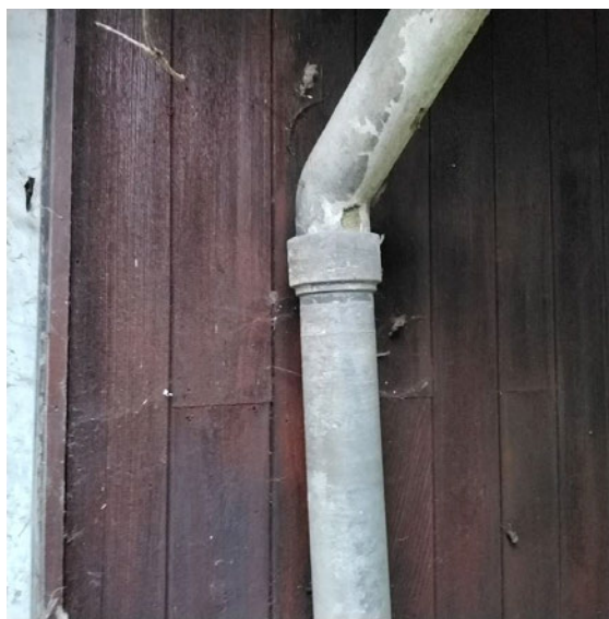
Sample 23: External. Exterior. Cement downpipes around perimeter
