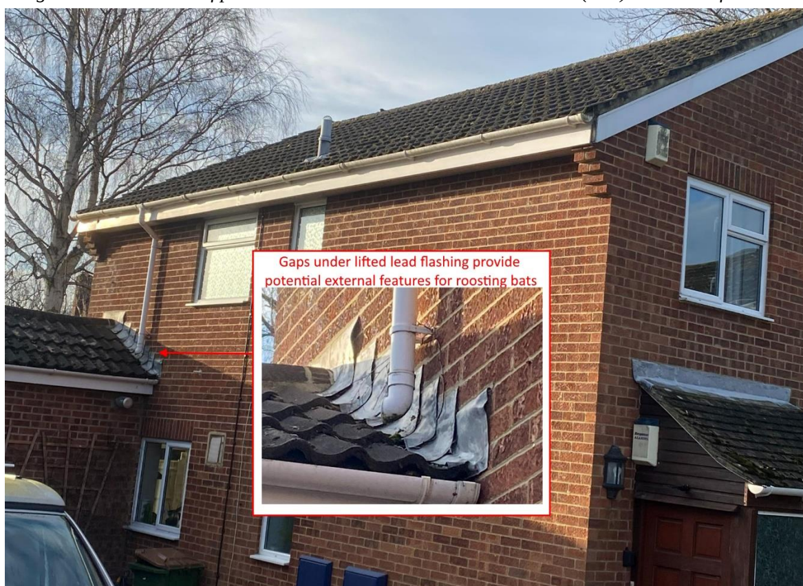
Image 4.3.1.1. Location of potential external roost locations on the east (side) elevation of the house.
