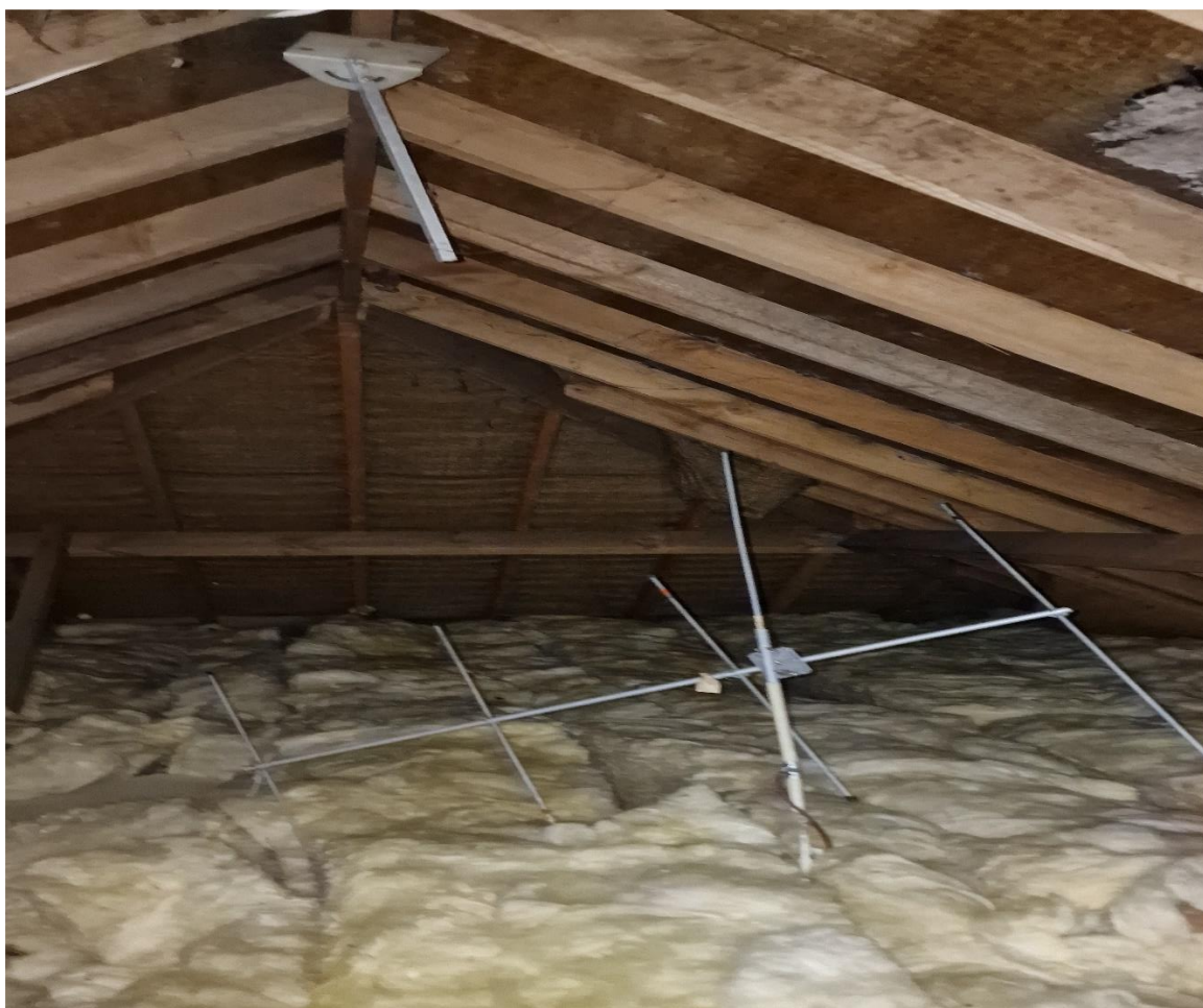
Picture 4: Showing the internal roof structure.
