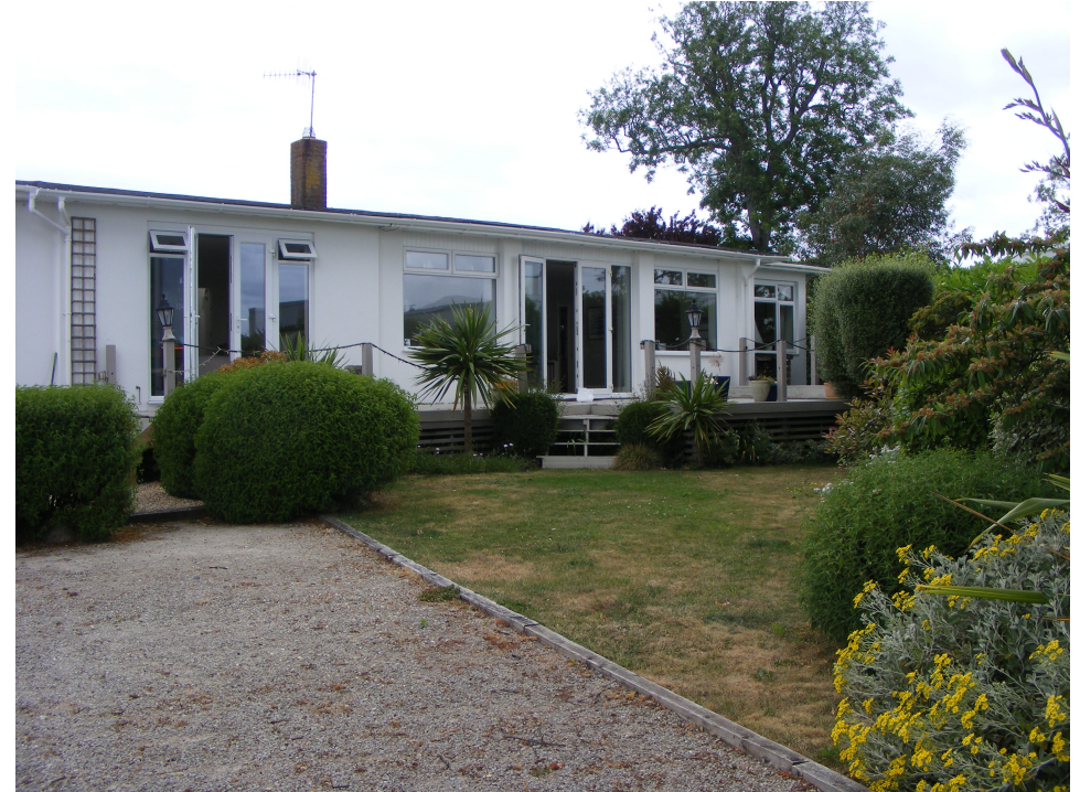
(06) Photo looking West from within No.15's rear garden at the remainder of the existing East Elevation, highlighting this elevations door and window opening configuration, due to be reconfigured within the current proposal. In addition, this photo also highlights the existing material character of the rear terrace, due to be replaced with a new paved terrace incorporating a glass balustrade, raised box planter and steps into the rear garden.
