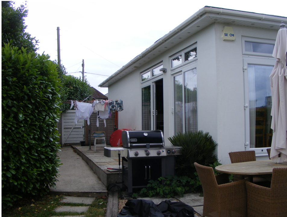
(07) Photo looking North-West along No.15's Southern boundary highlighting the area proposed for the small side extension, along with the configuration of varying ground level or patio level changes relative to the rear.
