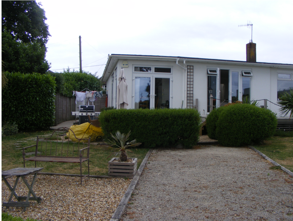
(05) Photo looking West from within No.15's rear garden, looking at the South-Eastern corner of the existing bungalow where a small side extension is proposed, creating space for the relocated kitchen and utility room, whilst offering access into retained and enlarged garage.
