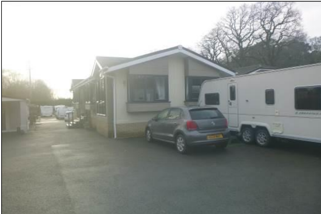
Photograph 2 Showing the amenity building and dwelling to the southeast
